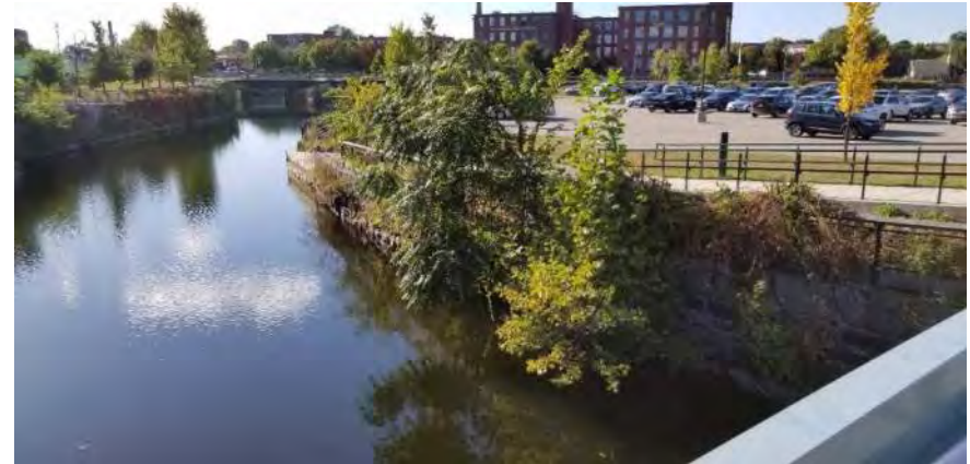
Polygon No.: 25 Photo No.: 25 Date: 9/25/2019 Direction Photo Taken: Northerly Description: The vegetation growing out of the canal wall includes one sycamore, several tree of heaven, glossy buckhorn, and ragweed.
