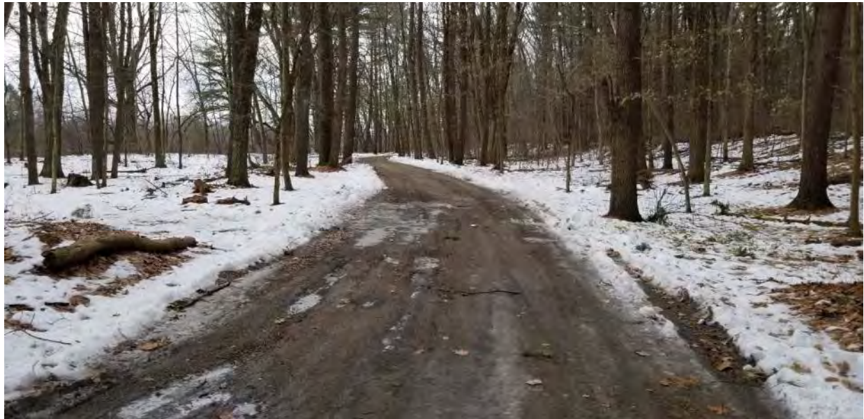
Photo 5 – Access road to Greeley Boat Ramp
