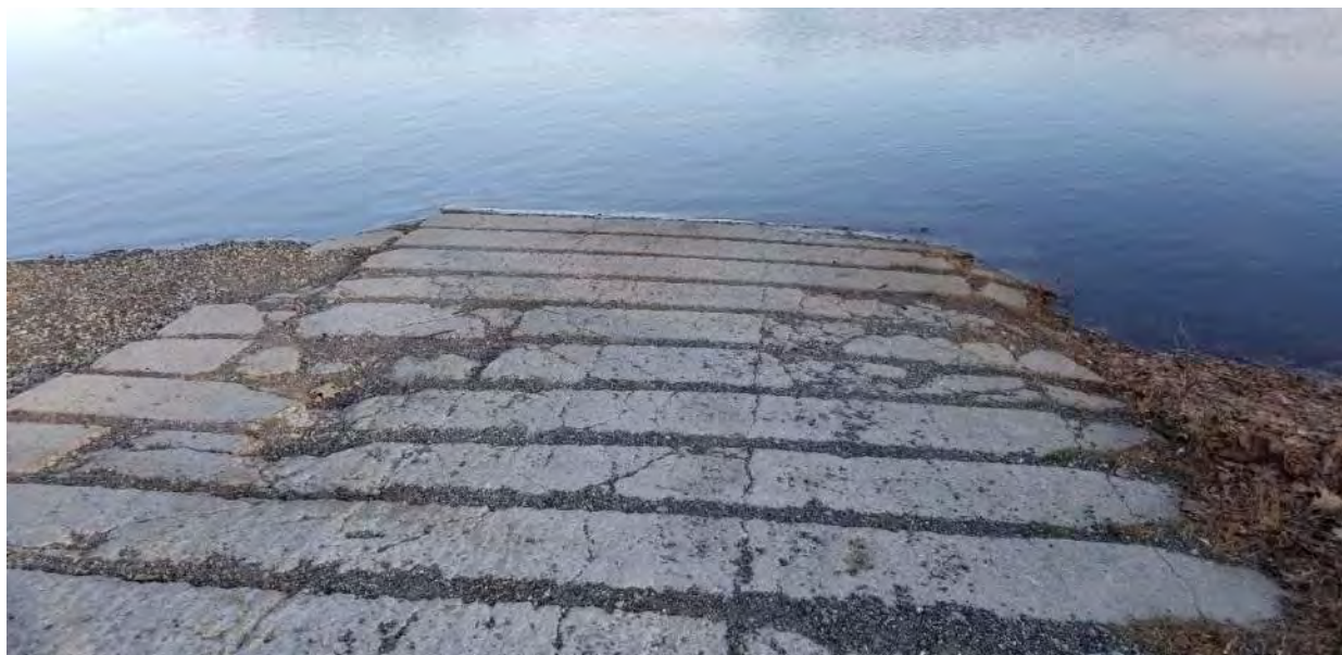
Photo 2 – Chelmsford Boat Access Ramp
