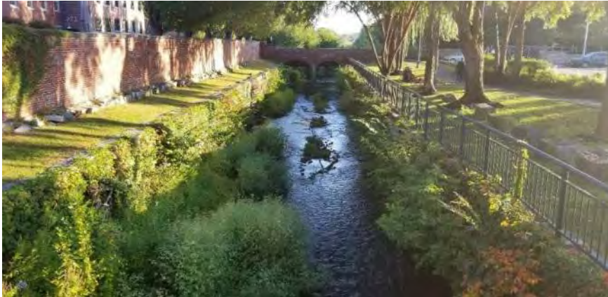
Polygon No.: 45 and 46 Photo No.: 45 Date: 9/26/2019 Direction Photo Taken: Northeasterly Description: Vegetation growing on the eastern side of the canal wall (left side of the photograph) includes several tree species (i.e. mulberry, buckthorn, tree of heaven, etc.) and dense vines, including Boston Ivy and poison ivy. Vegetation growing on the western side of the canal wall (right side of the photograph) includes less trees than the eastern side of the canal and similar vine species.
