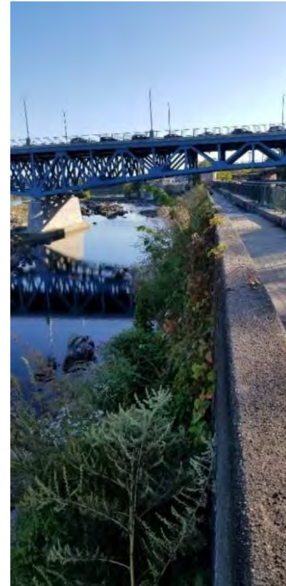
Polygon No.: 75 Photo No.: 75a Date: 9/27/2019 Direction: Northeasterly Description: Vegetation is growing from small sill under the first block down on the canal wall and is dominated by herbaceous plants such as ragweed, purple loosestrife, aster, scattered ferns, golden rod spp., scattered mulberry, elms, and buckthorn.
