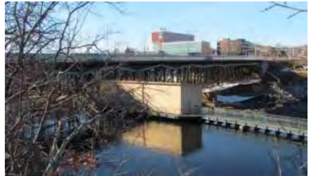
Northern Canal Wasteway Gatehouse (DCR)
