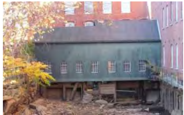
Boott Dam Gatehouse (DCR)
