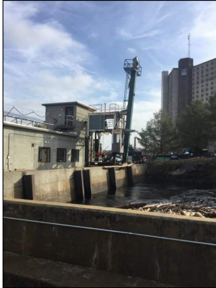
Figure E.7-36. E.L. Field Powerhouse with University of Massachusetts Lowell in the Background
