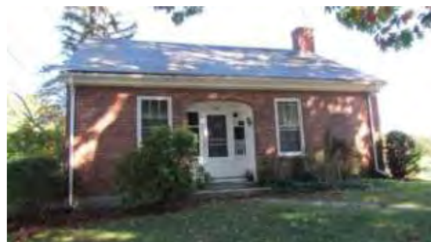
North Schoolhouse/Park HQ (DCR)
