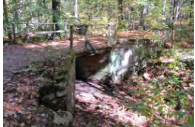
Small bridge on Woodchuck Trail (DCR)
