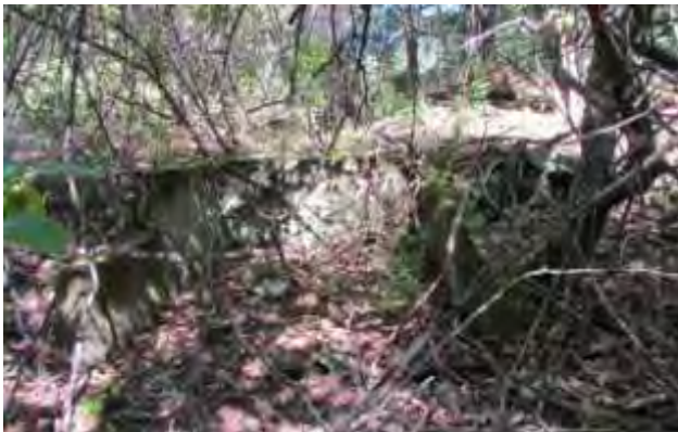
Outbuilding Foundation (DCR)
