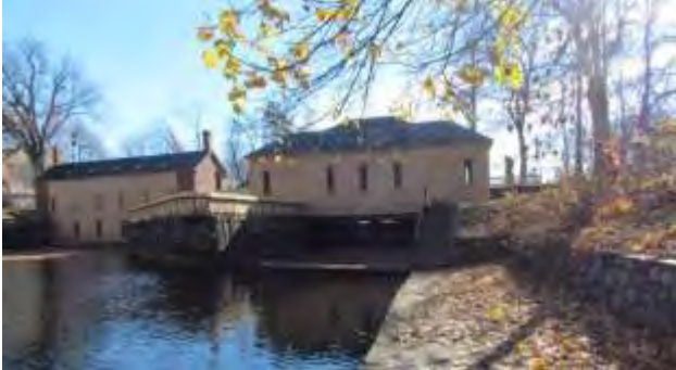
Guard Locks Gatehouse, left, and Guard Locks Lock House, right (DCR)
