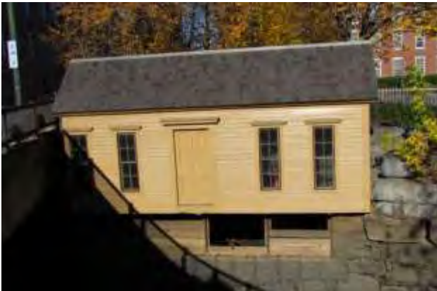
Massachusetts Wasteway Gatehouse (DCR)
