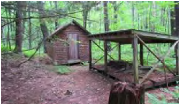
Cabin Shed and Lean-to (DCR)
