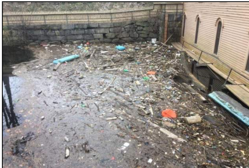
Figure E.7-37. Waterborne trash on the Pawtucket Canal at Guard Lock and Gates Facility.
