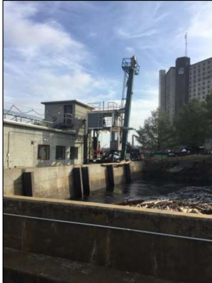
Figure E.7-36. E.L. Field Powerhouse with University of Massachusetts Lowell in the Background
