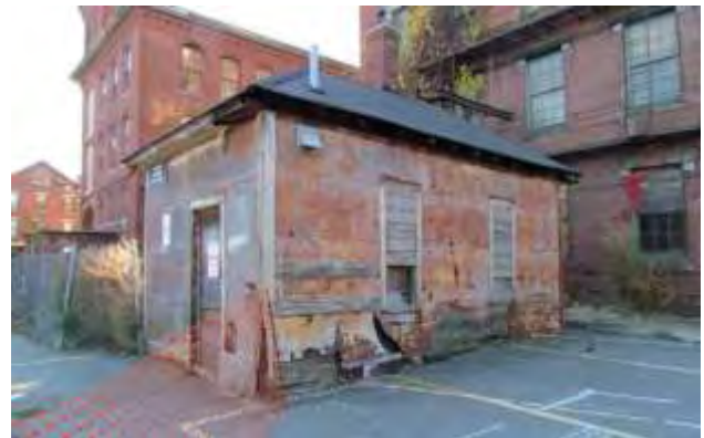
Hamilton Wasteway Gatehouse (DCR)
