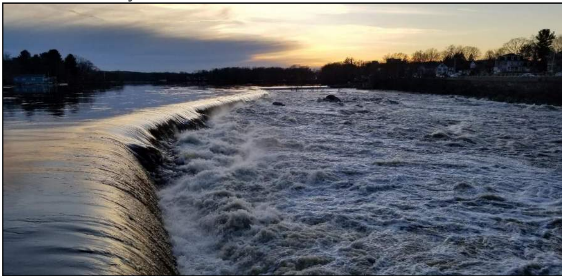
Figure E.7-35. Westerly View of Pawtucket Dam from the Pawtucket Gatehouse
