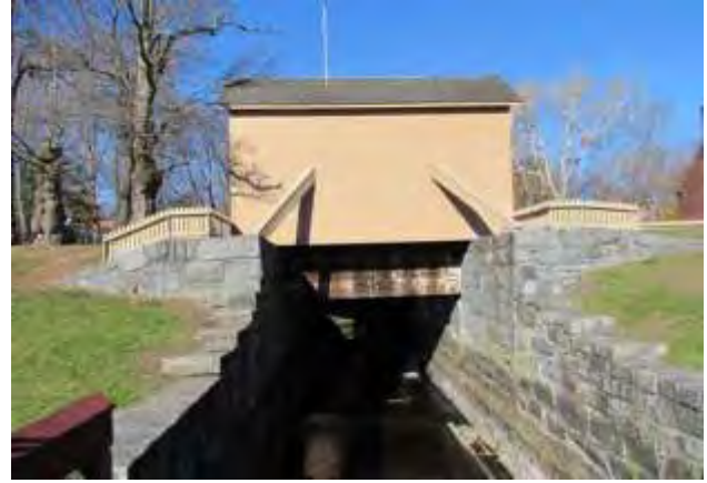
Great Gate and Gatehouse (DCR)
