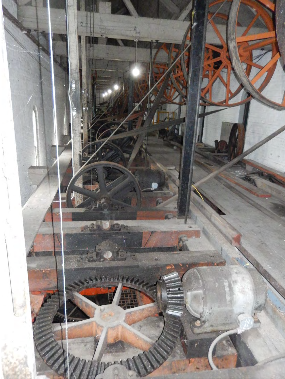
Figure 5-5. Pawtucket Gate House, belt-and-line shaft system with electric motor drive in foreground.
