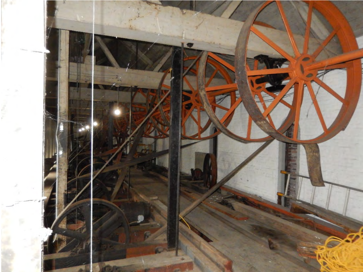
Figure 5-4. Pawtucket Gate House, belt-and-line shaft system.
