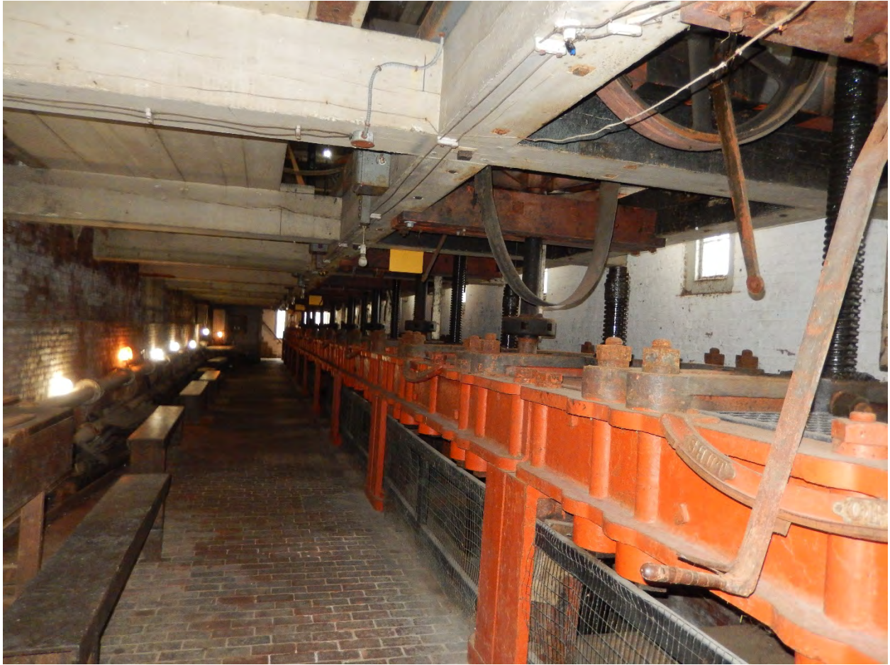
Figure 5-6. Pawtucket Gate House, sluice gate casings, with belt drives above.
