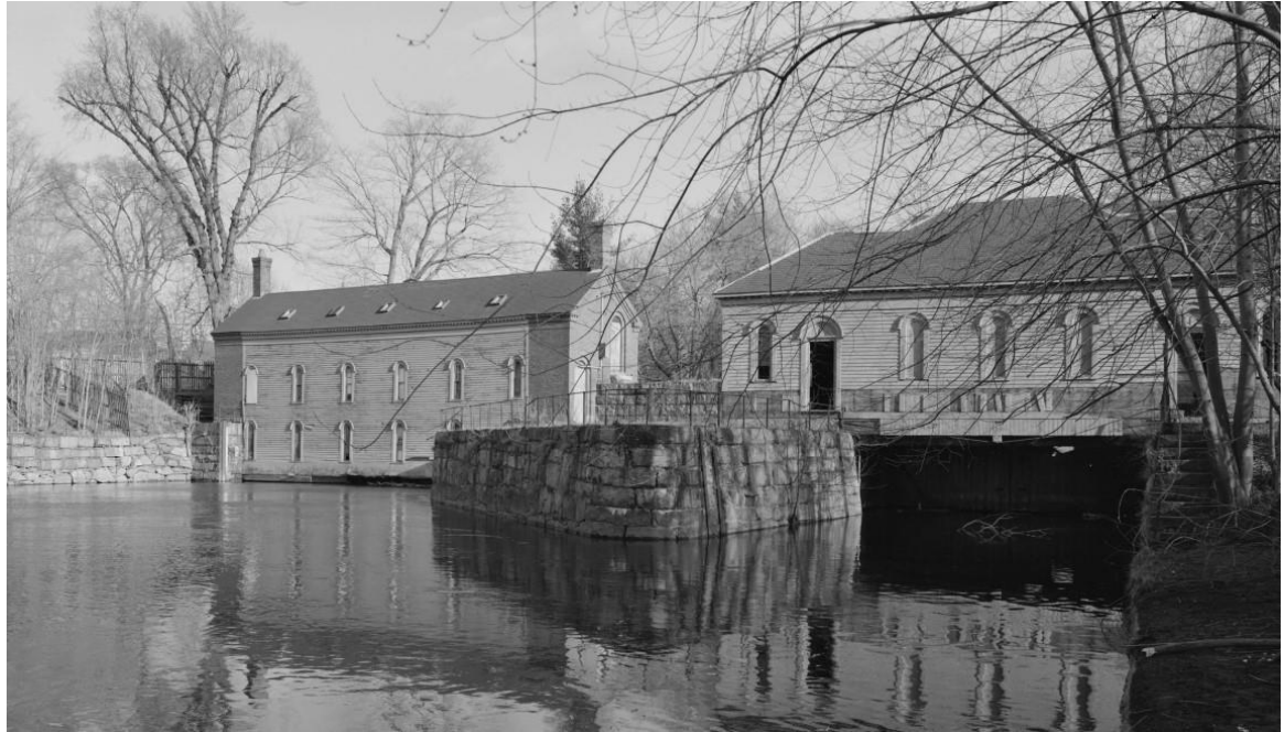
Photo 5-7. 1976 - Guard Lock and Gates Facility viewed from upstream. The Guard Gatehouse is on the left and the Lock Canal and Lock House are on the right.
