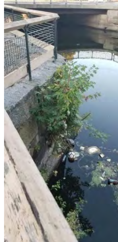
Vegetation Point No.: VP-11 Photo No.: VP-14 Date: 9/26/2019 Direction Photo Taken: Southwesterly Description: A small clump of silver maples are growing out of the canal wall.
