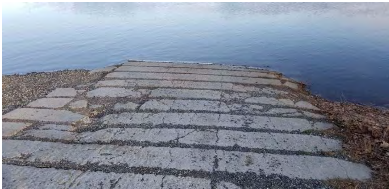
Photo 2 – Chelmsford Boat Access Ramp
