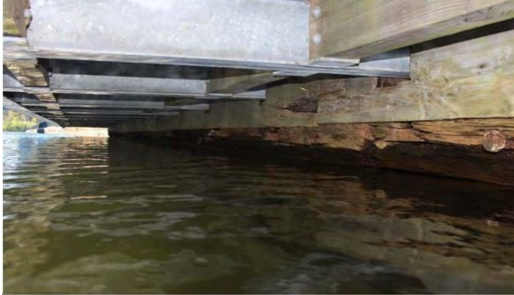
Photo 5-6. Northern Canal Waste Gatehouse underlying timber sill.
