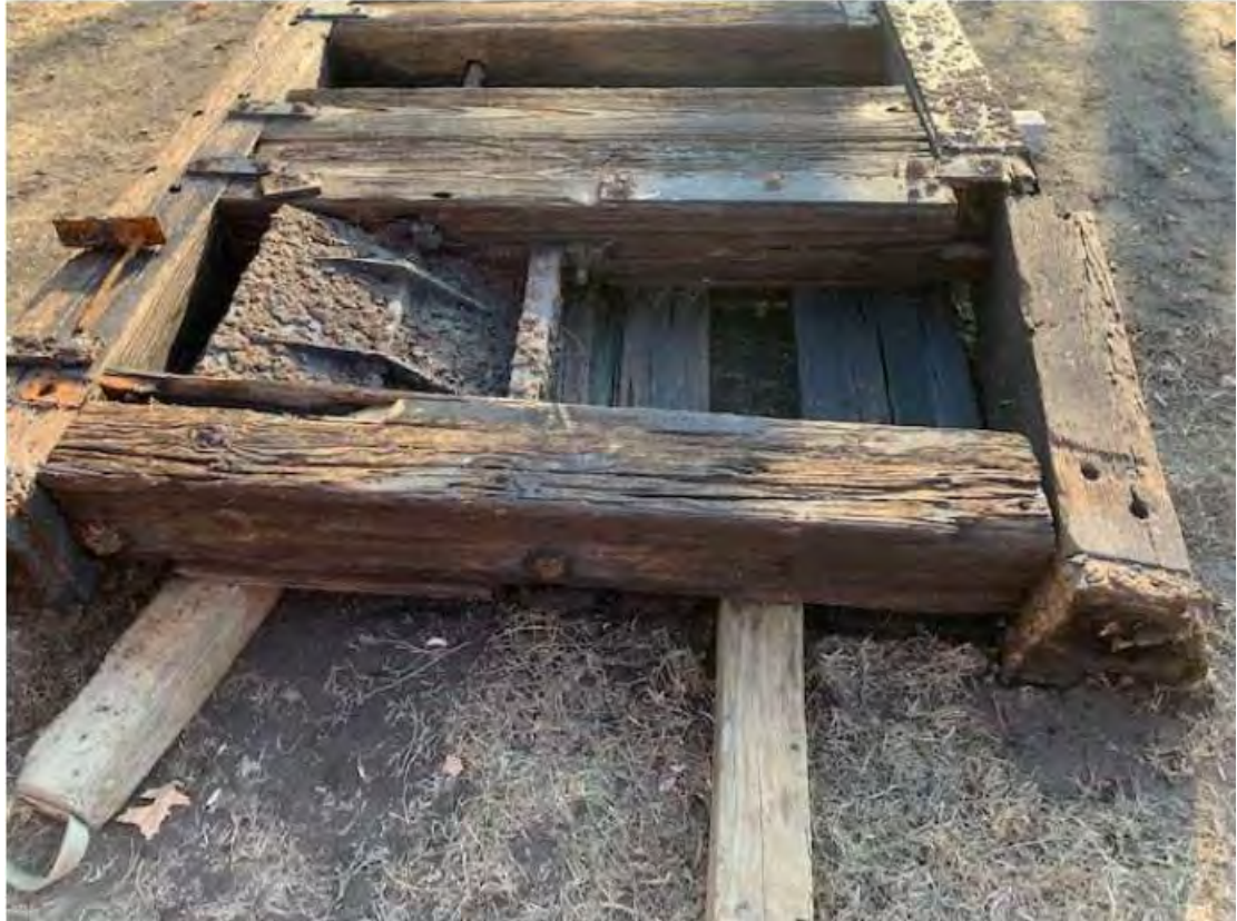
Photo 5-4. Photo of wear of submerged portion of the Northern Canal Gate removed for repair.
