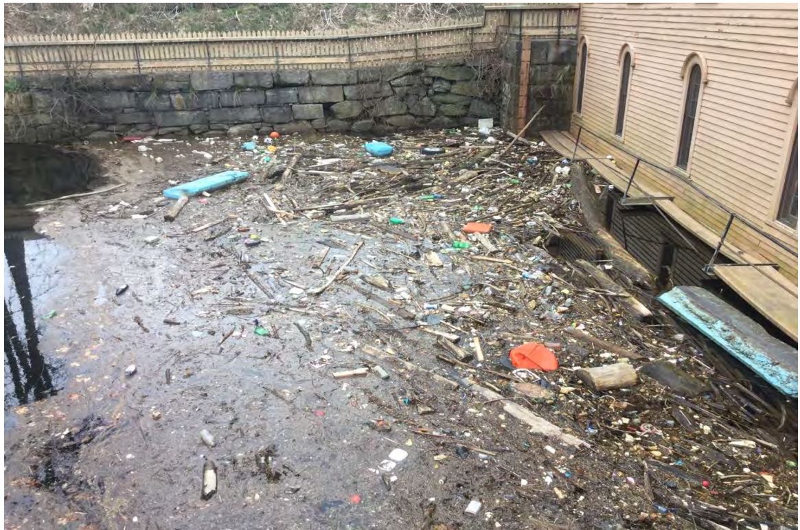
Photo 5-8. 2019 - Guard Lock and Gate Facility.
