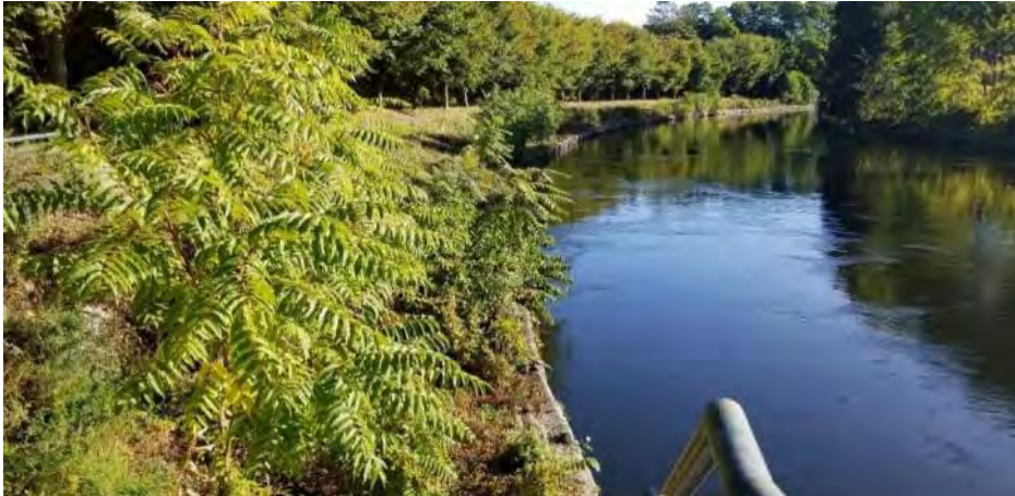
Polygon No.: 79 Photo No.: 79 Date: 9/27/2019 Direction Photo Taken: Northeasterly Description: Tree of heaven trees and vines are growing on top of the canal wall and within approximately 3 feet of the canal wall.
