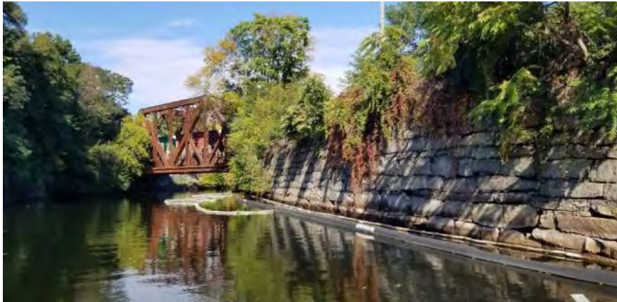
Polygon No.: 66 Photo No.: 66a Date: 9/26/2019 Direction Photo Taken: Northerly Description: The vegetation growing out of the eastern side of the canal wall (right side of the photograph), at the top of the wall, includes trees, such as tree of heaven and birch, and vines, such as Boston ivy.
