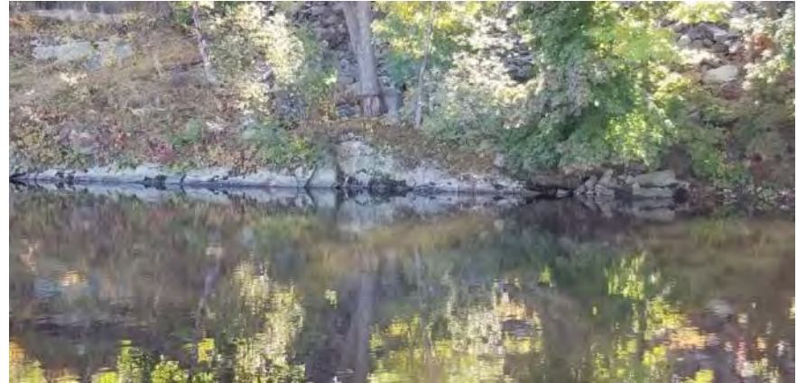
Polygon No.: 93 Photo Location No.: P-10 Date: 9/27/2019 Direction Photo Taken: Southerly Description: Vegetation is growing on bedrock along south side of the canal.
