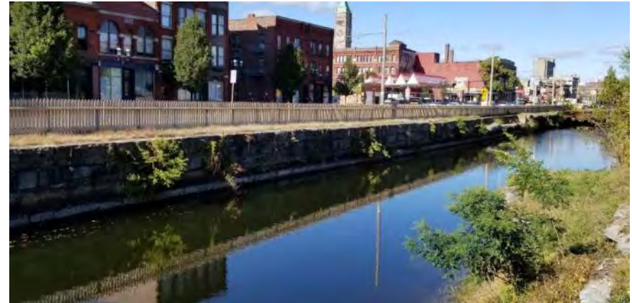
Polygon No.: 16 Photo No.: 16 Date: 9/25/2019 Direction Photo Taken: Northerly Description: Approximately 20 percent of the canal wall has woody trees (i.e. elms, locust, and mulberry) or herbaceous plants growing on it.
