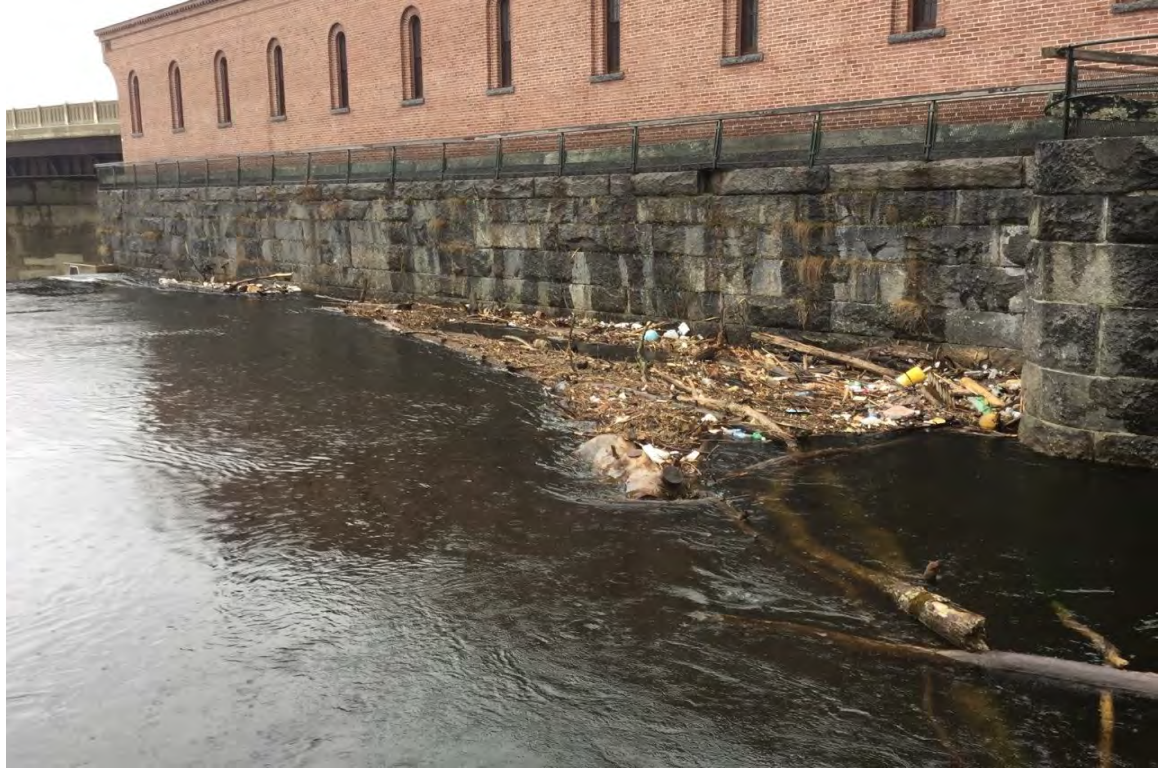
Photo 5-1. Northern Canal Lock and Pawtucket Gatehouse.
