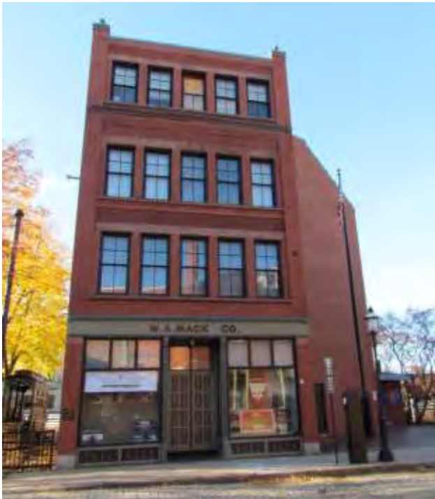
The Mack building, prior to the window replacement project. (DCR)
