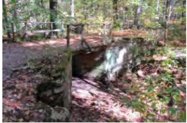
Small bridge on Woodchuck Trail (DCR)
