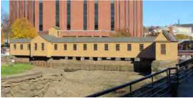
Lower Locks Gatehouse and Watch House (DCR)
