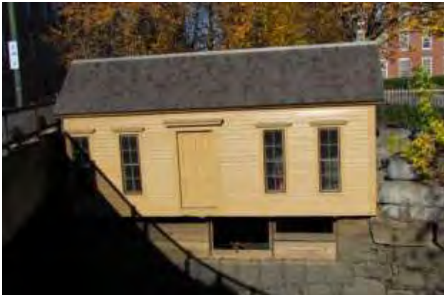
Massachusetts Wasteway Gatehouse (DCR)
