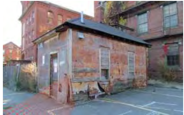
Hamilton Wasteway Gatehouse (DCR)
