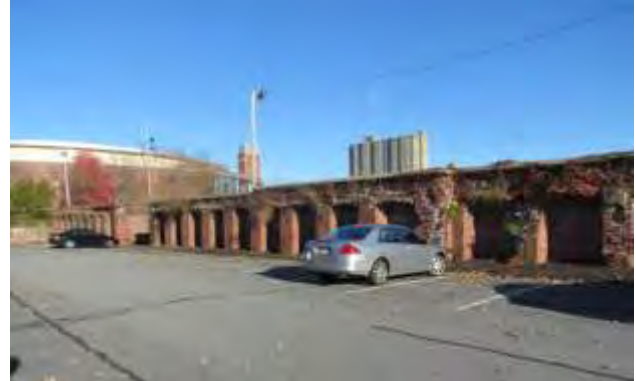
The eastern section of the wall in Tremont Yard. (DCR)
