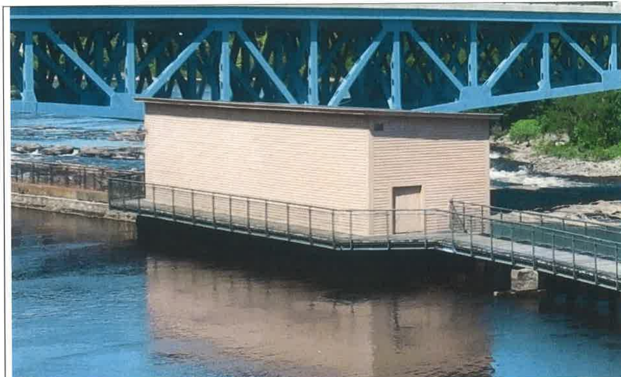
Photograph 1 – Northern Canal Waste Gatehouse, viewed from the southeast.
