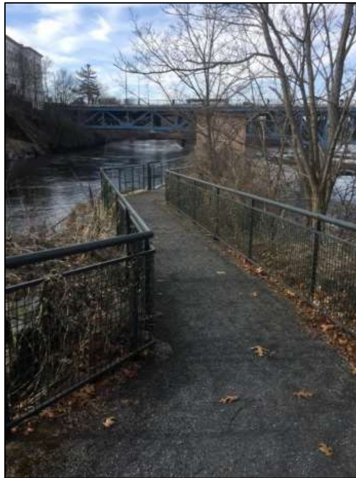
Figure E.7-31. Pedestrian Walk with View of the Northern Canal (left) and Bypass Reach (right).
