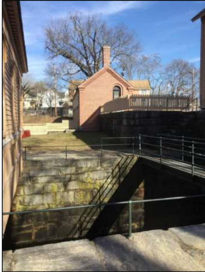
Figure E.7-32. Guard Lock and Gates Facility.
