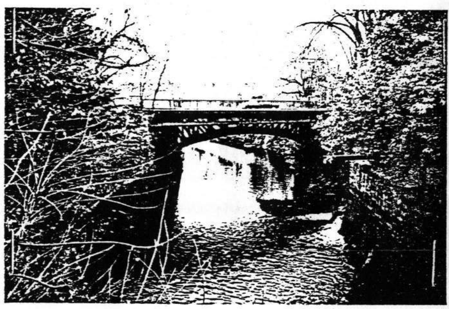
VIEW FROM north PHOTO TAKEN October 1979
