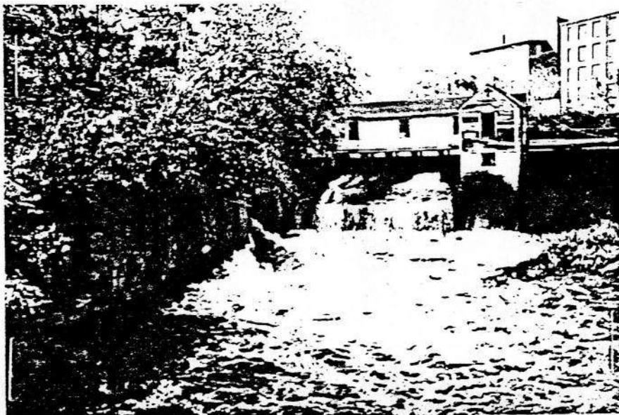
Detail of the Swamp Locks Dam (right) and lock (left), as seen from the east. Photo taken in August 1979.
