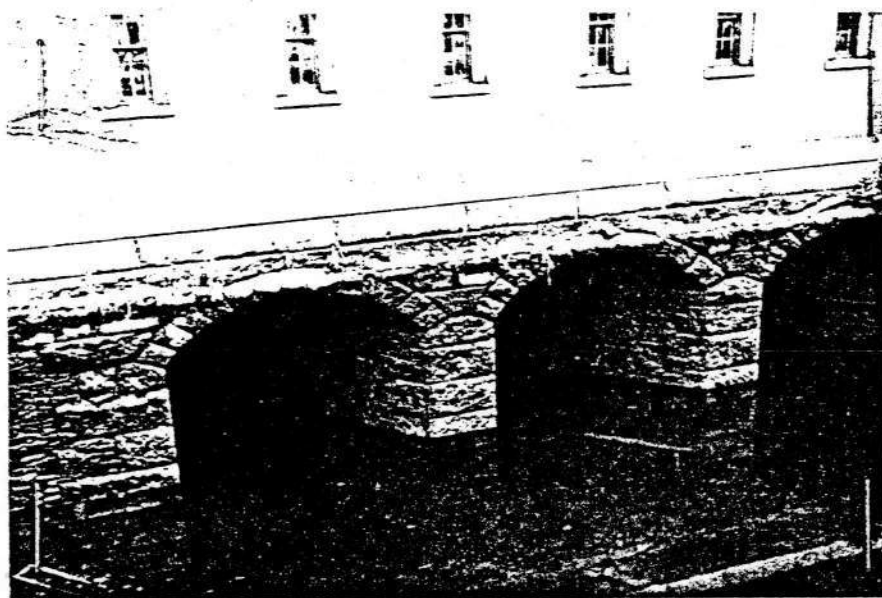
Detail of the arches beneath the Merrimack Gate House. The Feeder extends toward the Canal perpendicularly, but the final arches meet the Canal at an acute angle, to reduce the turbulence of the merging courses of water. Photograph taken in November 1979.
