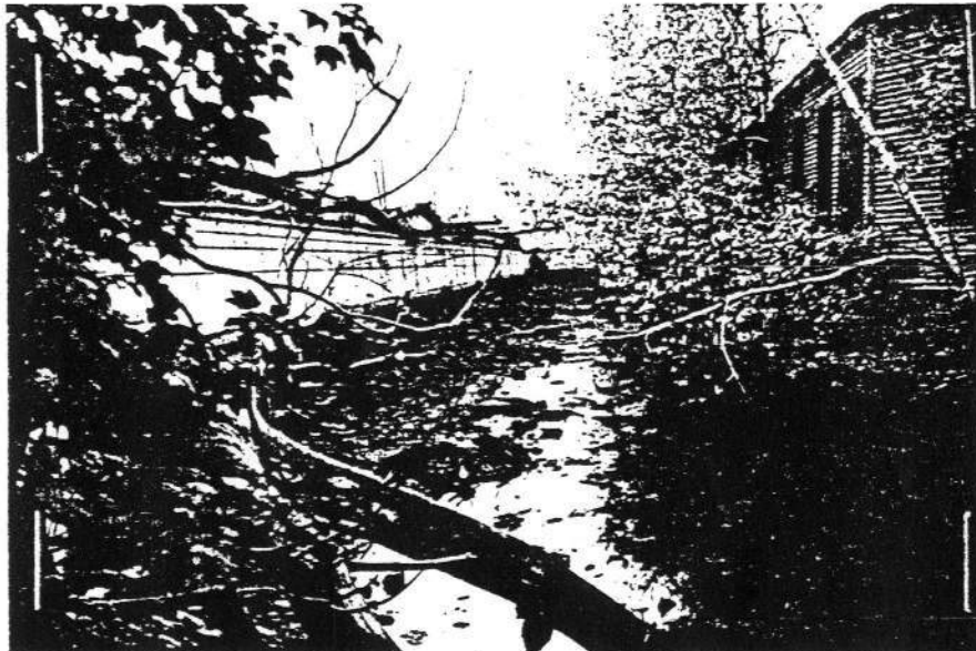
The Western Canal along lower Suffolk Street, as seen from the southwest. Note the poured concrete wall on the left. Photo taken in October 1979.
