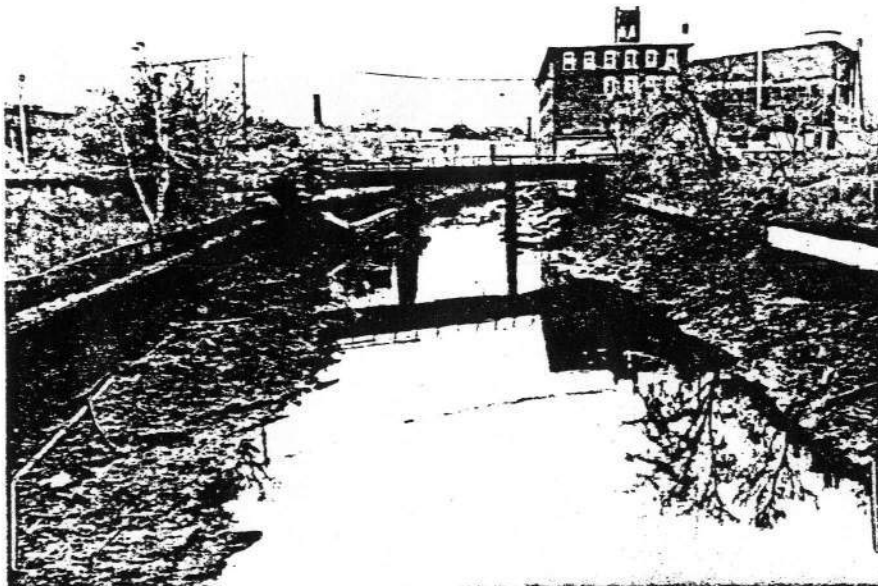
View from Thorndike Street west along the Pawtucket, showing the canal with most of the water drawn off. Photo taken in October 1979.
