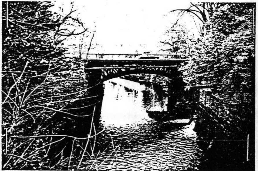
VIEW FROM north PHOTO TAKEN October 1979
