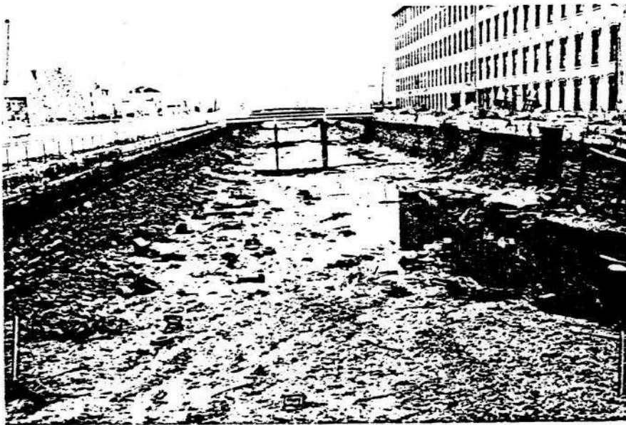
View from the southeast of the Northern Canal opposite the Suffolk millyard. Note the breadth of this canal. At right are Suffolk's penstock openings. Photo taken in October 1979.
