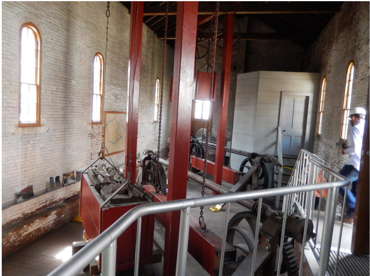
Figure 6-1. Moody Street Gate House, gate hoisting mechanisms.
