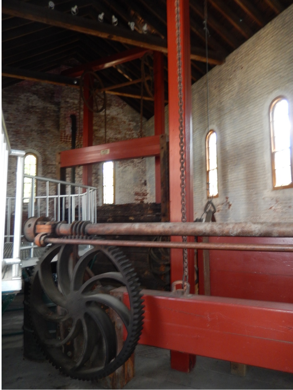
Figure 6-2. Moody Street Gate House, detail of gate hoisting mechanism
