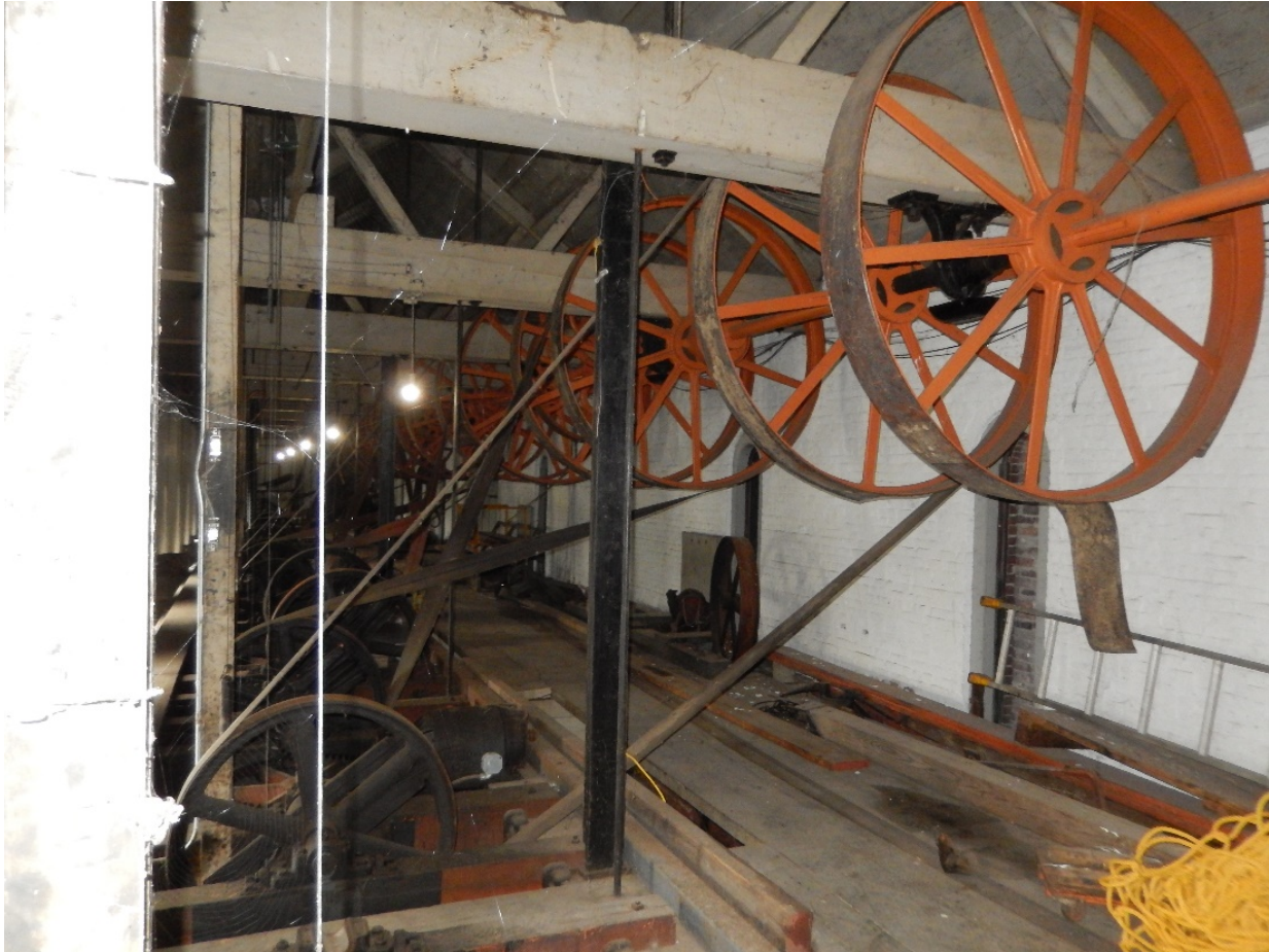
Figure 5-4. Pawtucket Gate House, belt-and-line shaft system.
