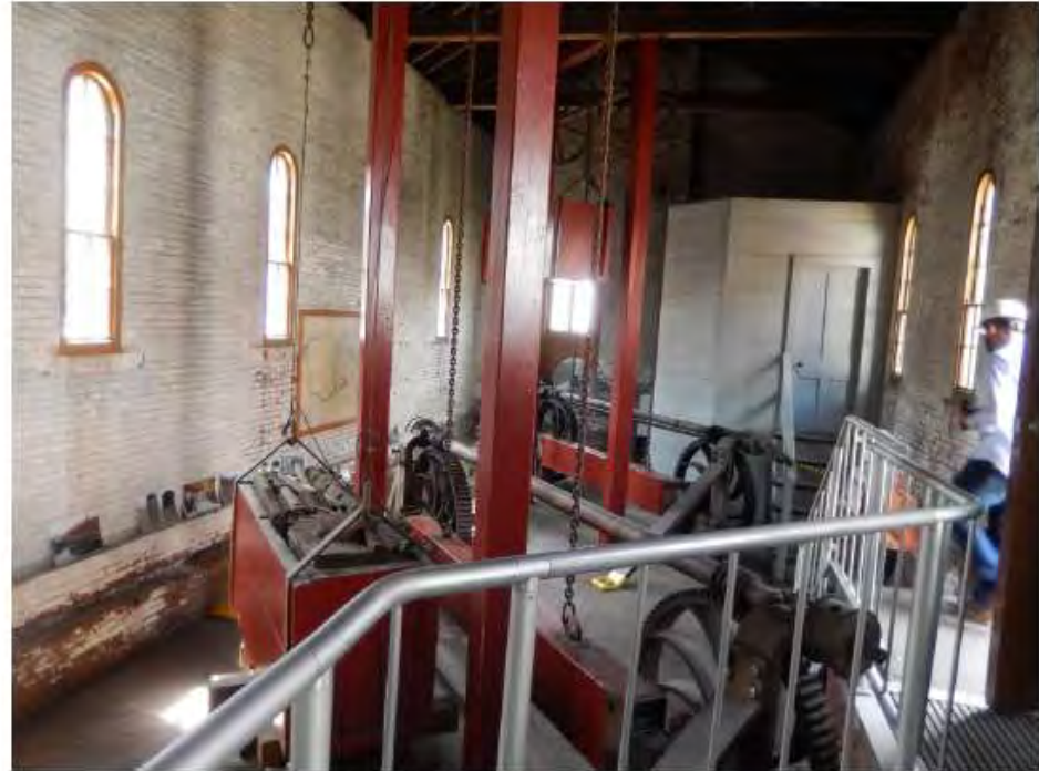
Figure 6-1. Moody Street Gate House, gate hoisting mechanisms.
