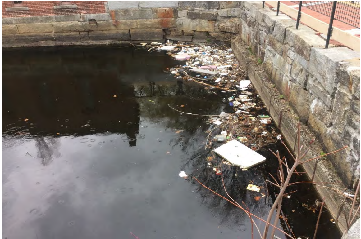
Photo 5-4. Waterborne trash on the Western Canal at the Northern Canal Junction.
