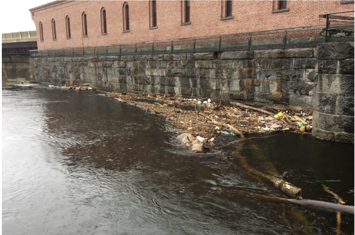
Photo 5-1. Waterborne trash on the Merrimack River upstream of the Northern Canal Gate entrance.
