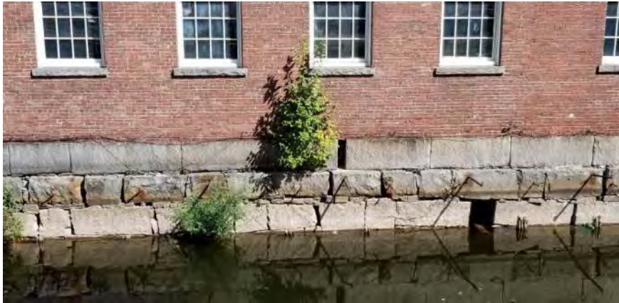
Vegetation Point No.: VP-1 Photo No.: VP-4 Date: 9/25/2019 Direction Photo Taken: Northeasterly Description: Vegetation includes a single shrub growing out of the canal wall below the brick building and sparse herbaceous species.
