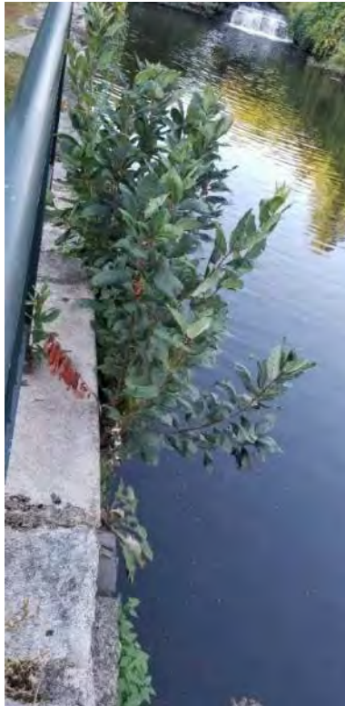
Vegetation Point No.: VP-14 Photo No.: VP-17 Date: 9/26/2019 Direction Photo Taken: Southwesterly Description: A small clump of shrubs growing out of the canal wall.
