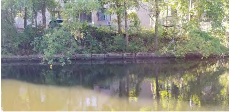
Polygon No.: 92 Photo No.: P-9 Date: 9/27/2019 Direction Photo Taken: Southerly Description: Vegetation growing on top of single stone/block wall on south side of the canal is forested habitat.
