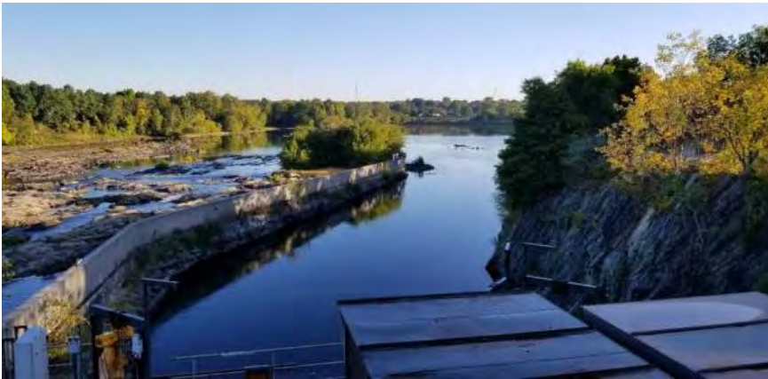
Photo Location No.: P-7 Date: 9/26/2019 Direction Photo Taken: Northeasterly Description: View from E.L. Field Powerhouse deck.
