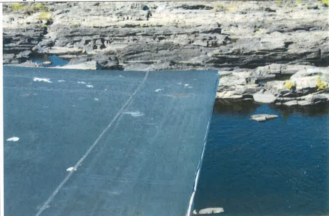
Photograph 2 – Delaminated edge of roof membrane at northeast corner of roof.
