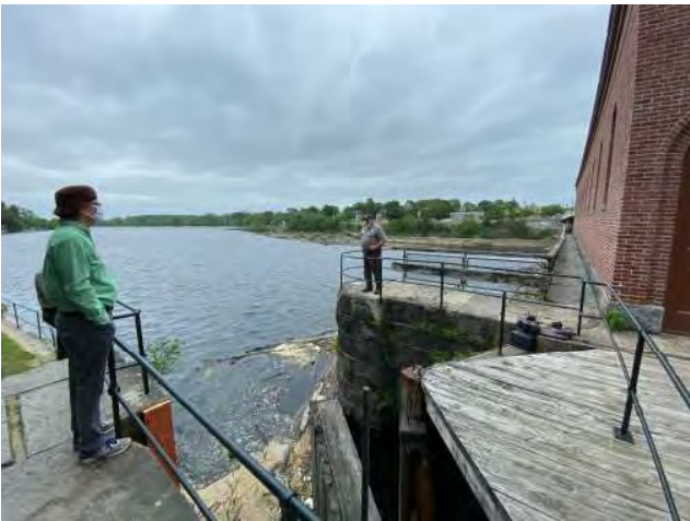
PHOTO 15: NORTHERN CANAL GATEHOUSE - LOCK CHAMBER GATES
