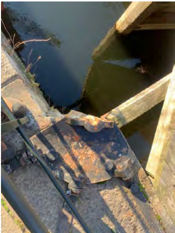
PHOTO 13: NORTHERN CANAL GATEHOUSE - LOCK CHAMBER GATES
