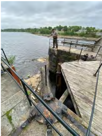
PHOTO 16: NORTHERN CANAL GATEHOUSE - LOCK CHAMBER GATES
