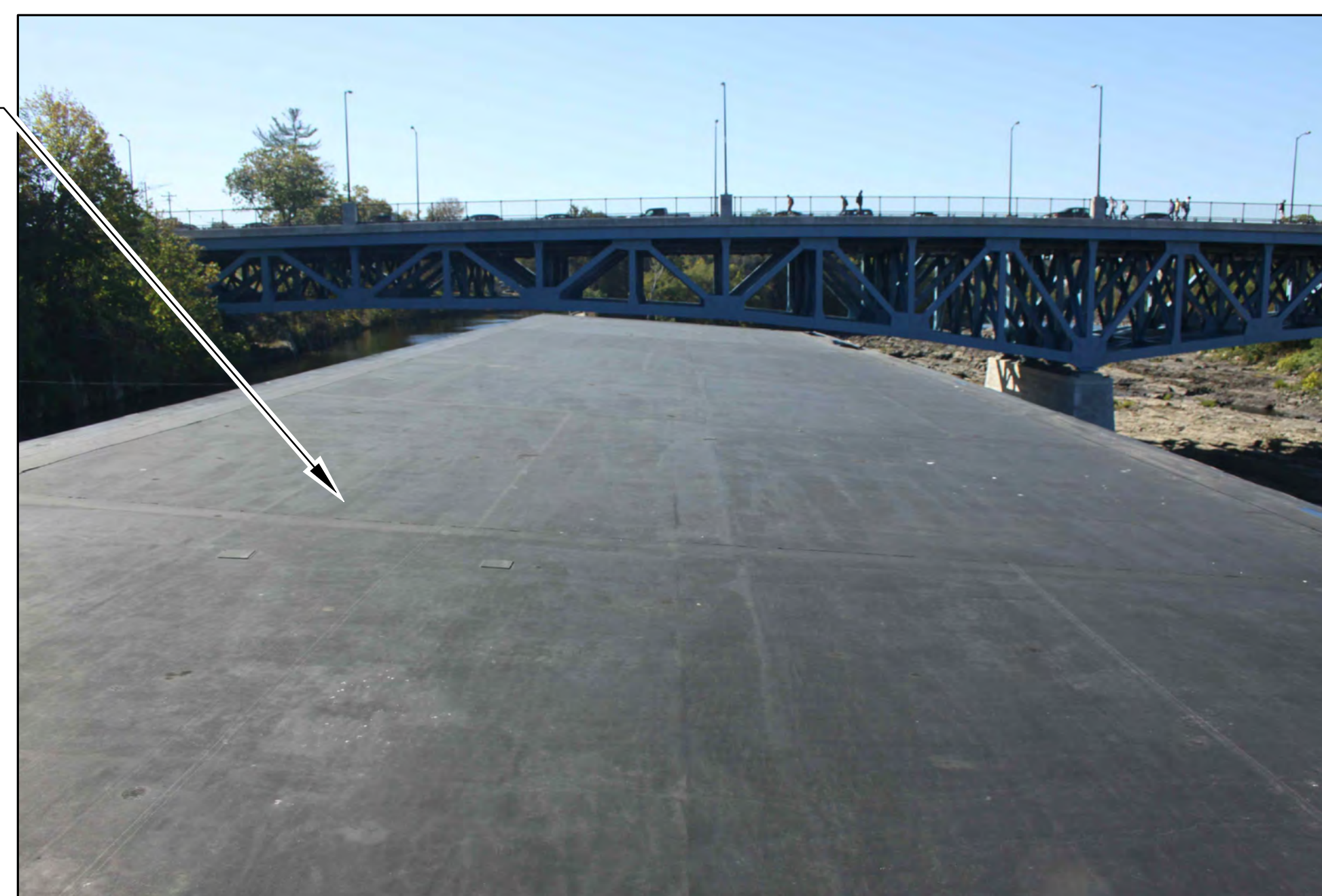
5 PHOTO 5 @ ROOF LOOKING WEST A4
