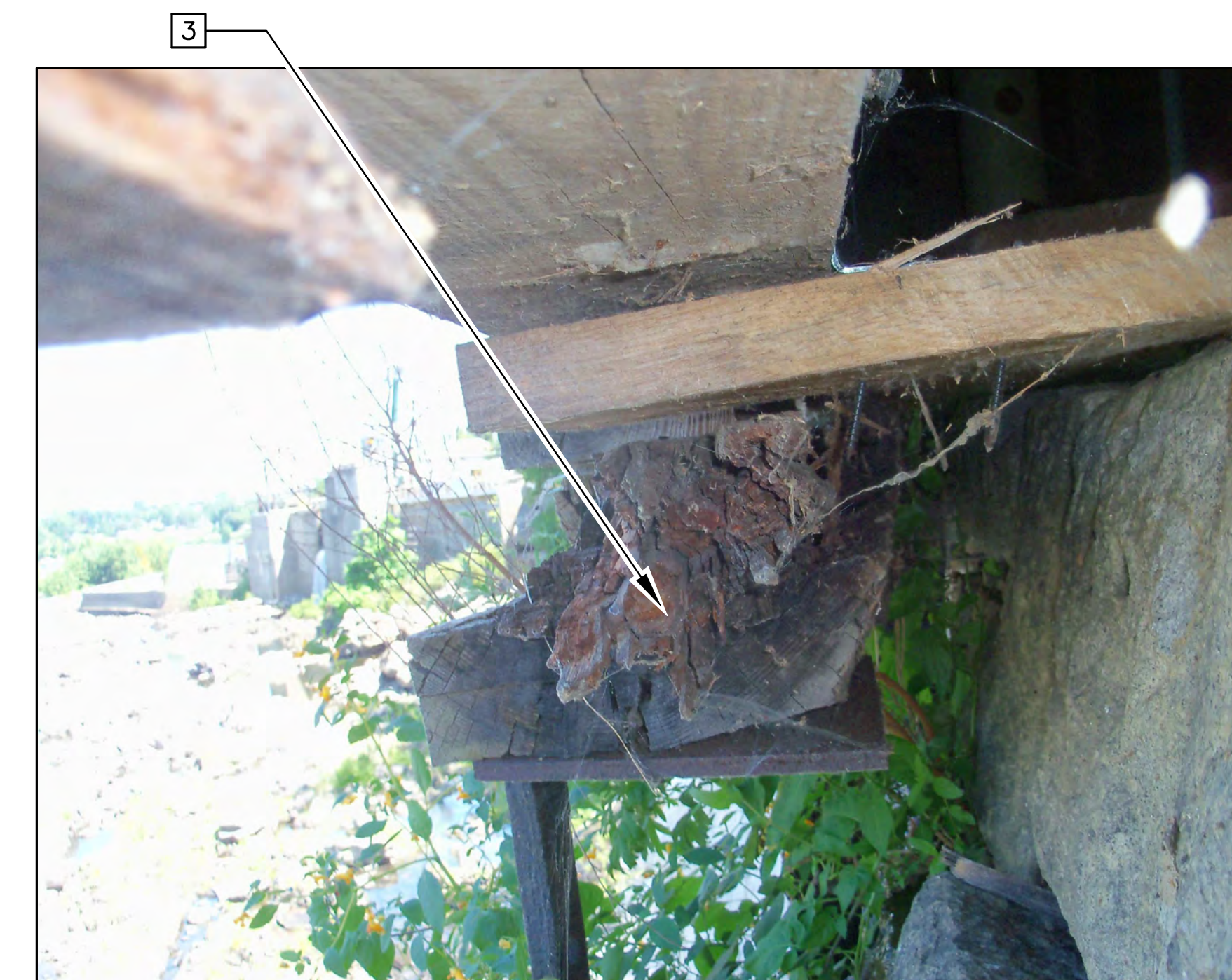
3 PHOTO 3 @ SILL UNDER NORTH WALL A4
