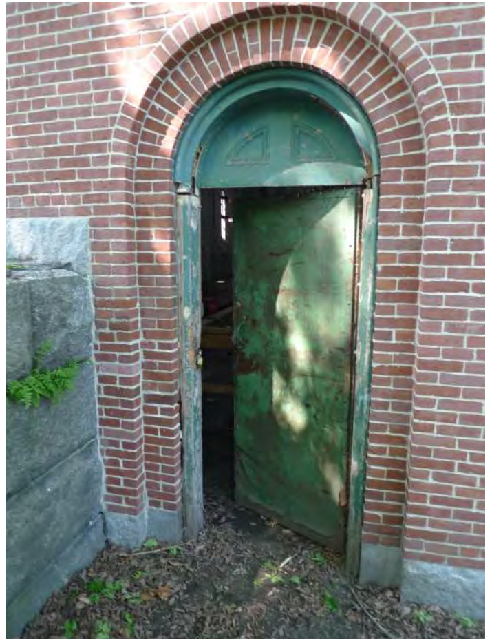
PHOTO 07: DETAIL AT LOWER GATEHOUSE DOOR
