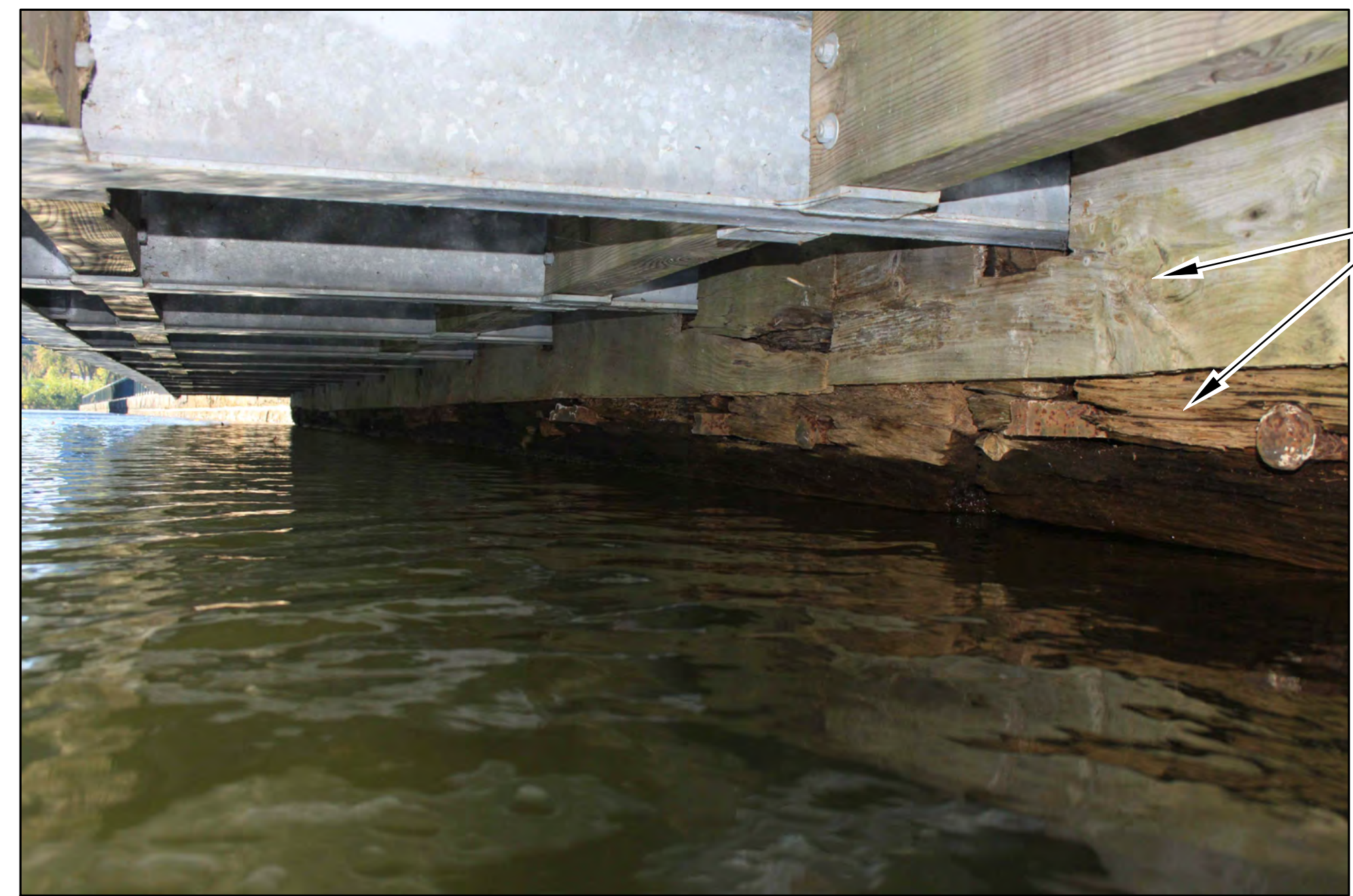
7 PHOTO 7 @ UNDERSIDE OF WALKWAY LOOKING WEST A5
