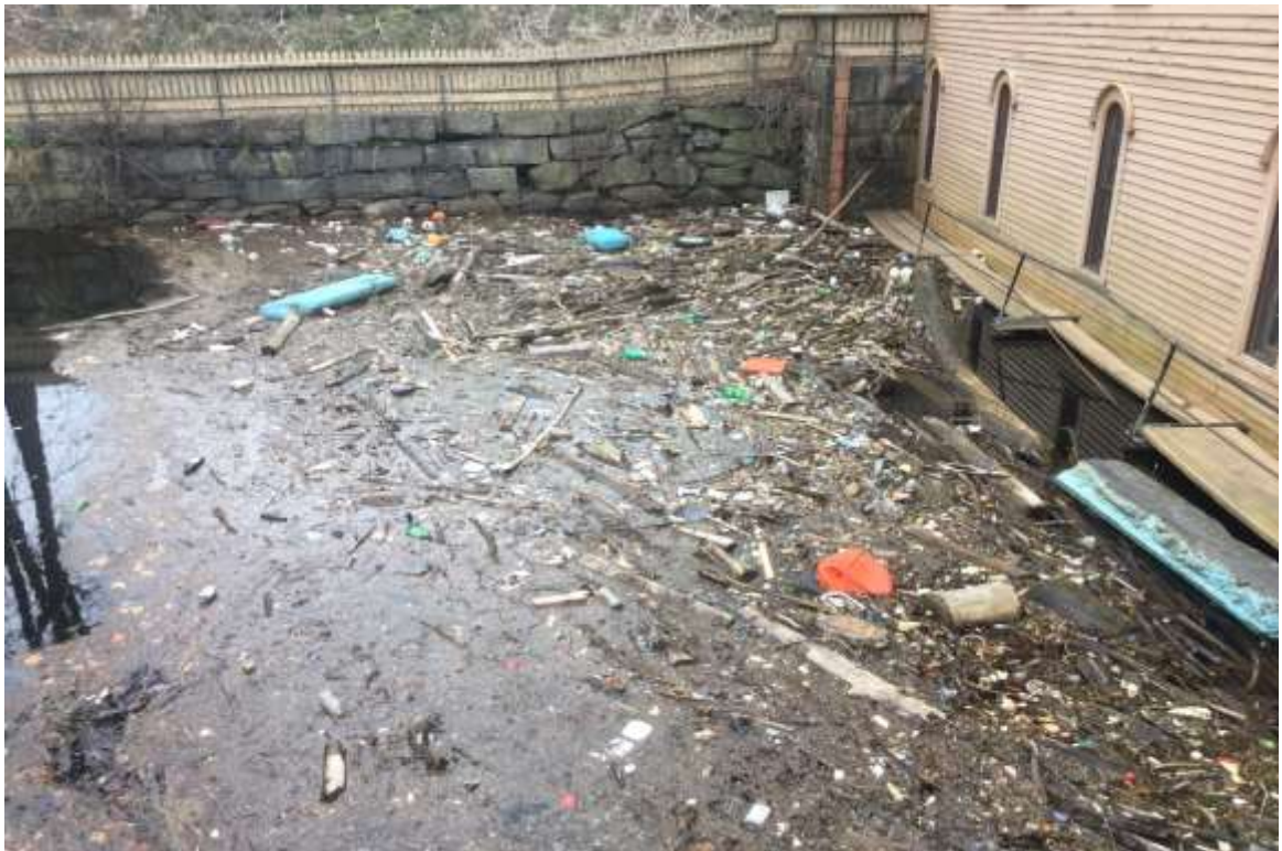
Photo 5-8. 2019 - Guard Lock and Gate Facility.
