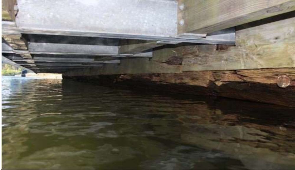
Photo 5-6. Northern Canal Waste Gatehouse underlying timber sill.
