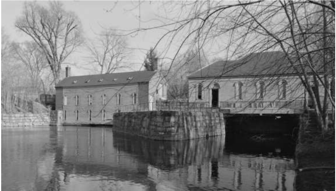
Photo 5-7. 1976 - Guard Lock and Gates Facility viewed from upstream. The Guard Gatehouse is on the left and the Lock Canal and Lock House are on the right.
