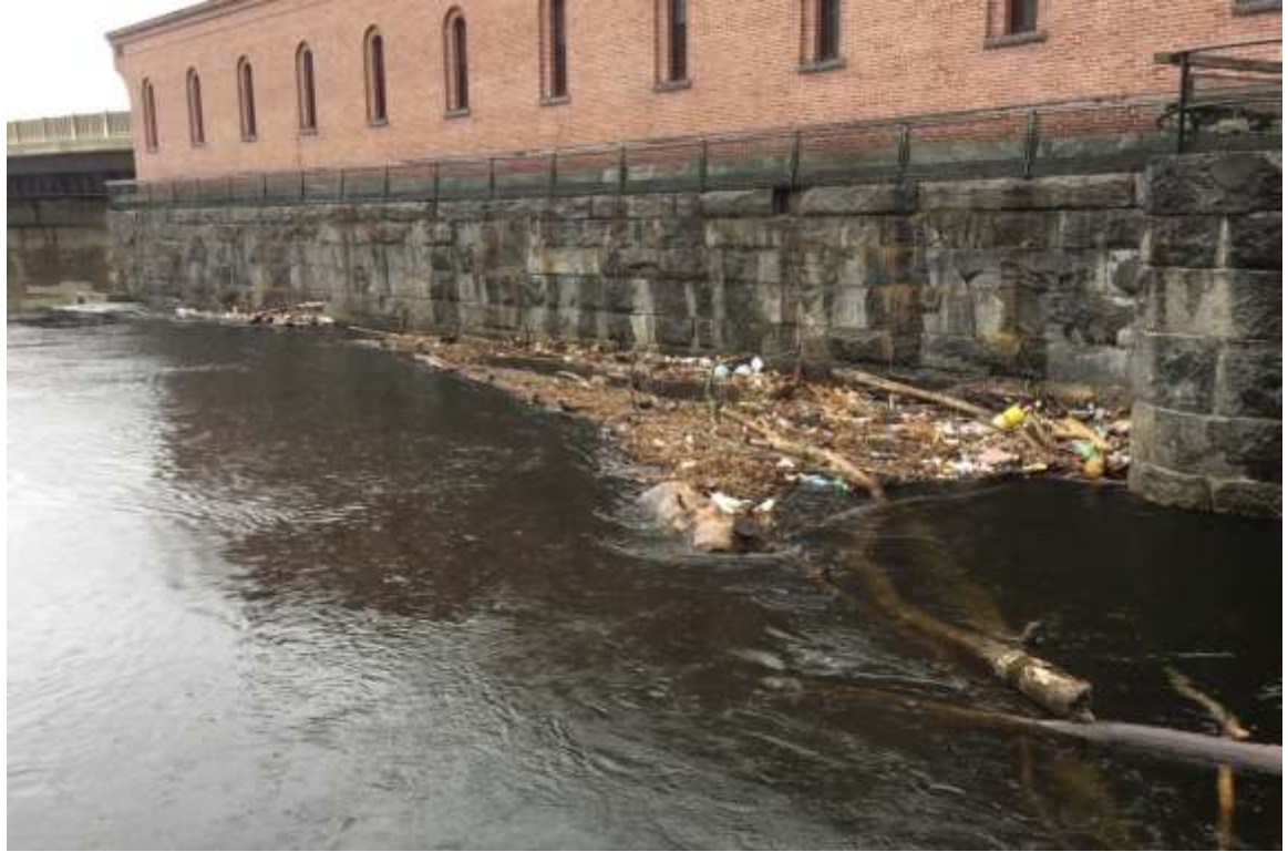
Photo 5-1. Northern Canal Lock and Pawtucket Gatehouse.
