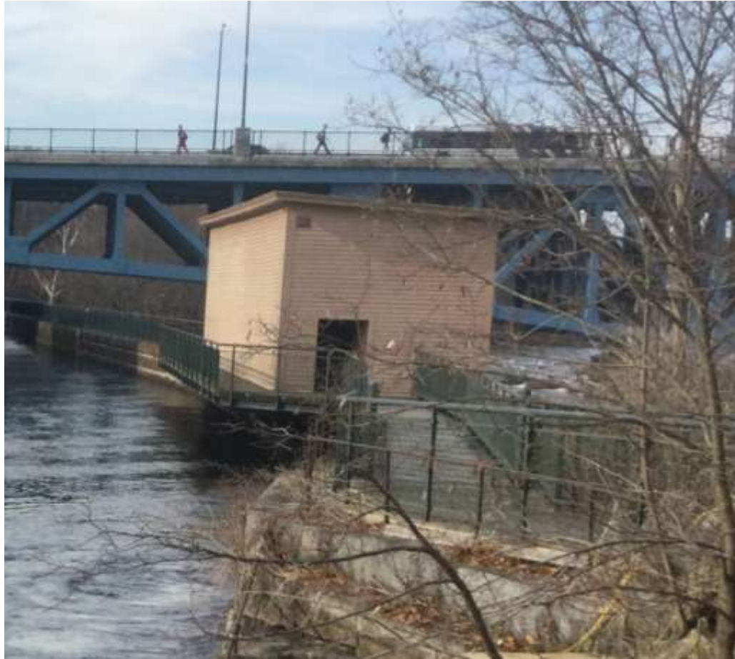
Photo 5-5. Northern Canal Waste Gatehouse atop the Northern Canal.
