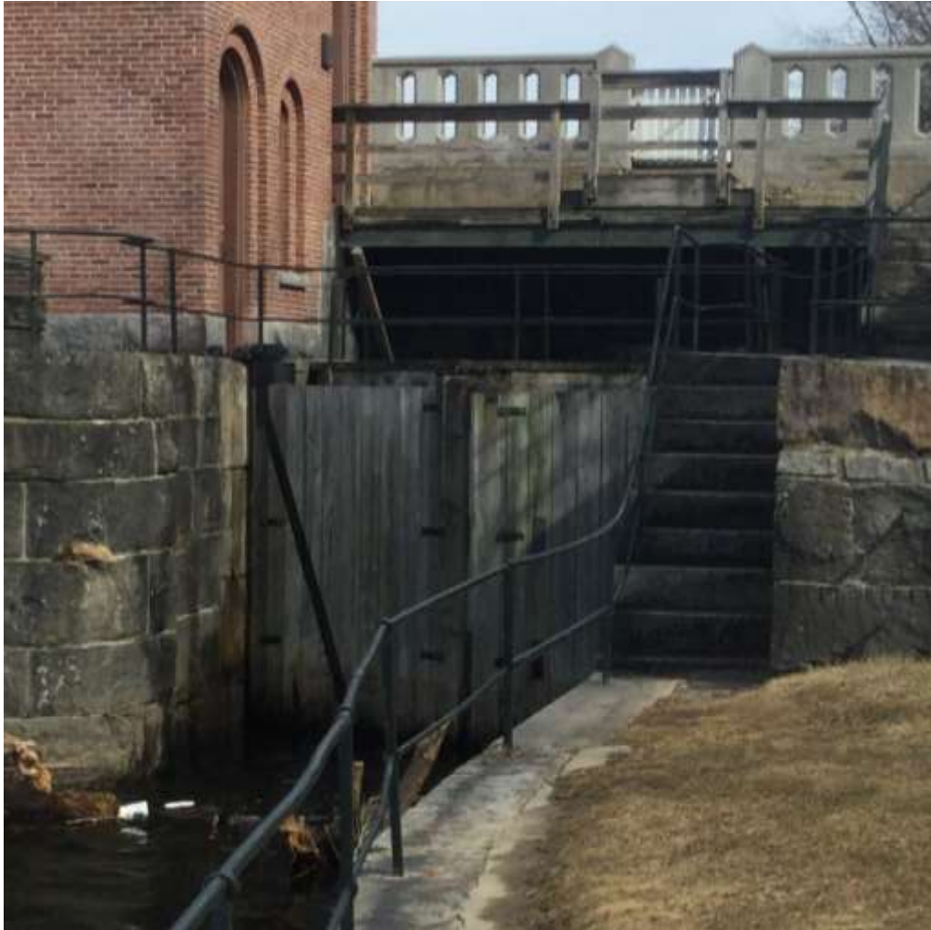
Photo 5-2. Pawtucket Gatehouse at Northern Canal Gate entrance (prior to 2018 gate damage).
