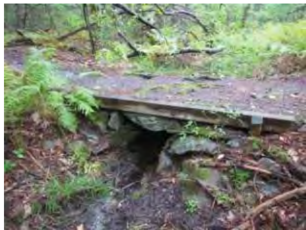
Stone Slab Bridge (DCR)
