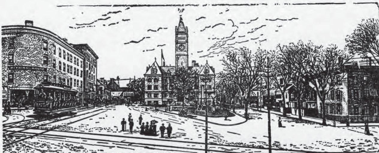
Figure 4-1 View of Monument Square from the east, ca. 1895.
