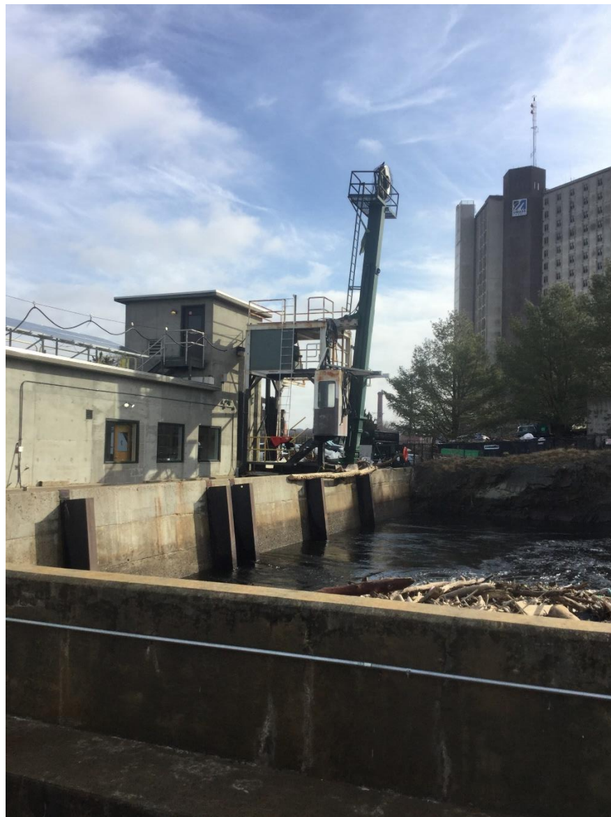
Figure 5.9-5. E.L. Field Powerhouse with University of Massachusetts Lowell in the Background.
