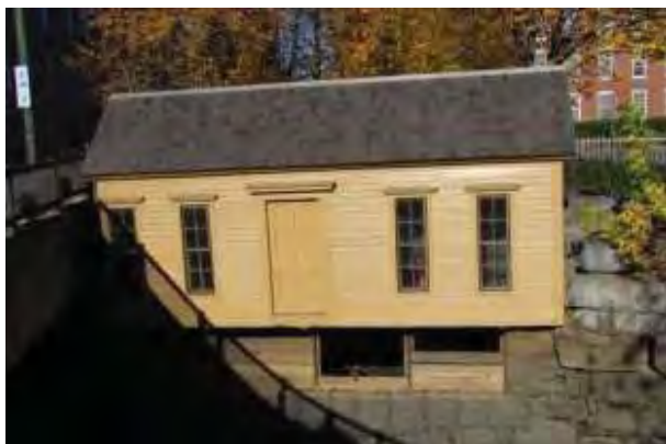
Massachusetts Wasteway Gatehouse (DCR)
