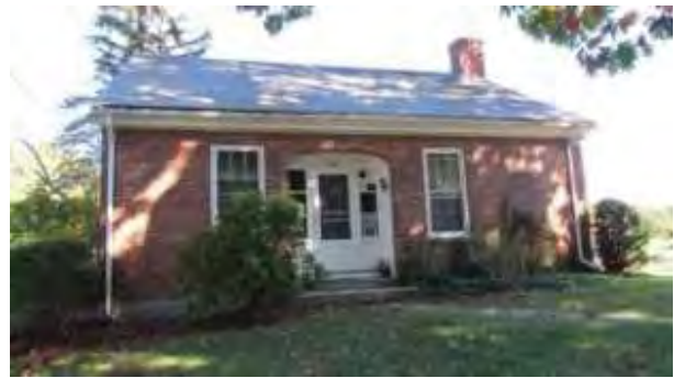
North Schoolhouse/Park HQ (DCR)
