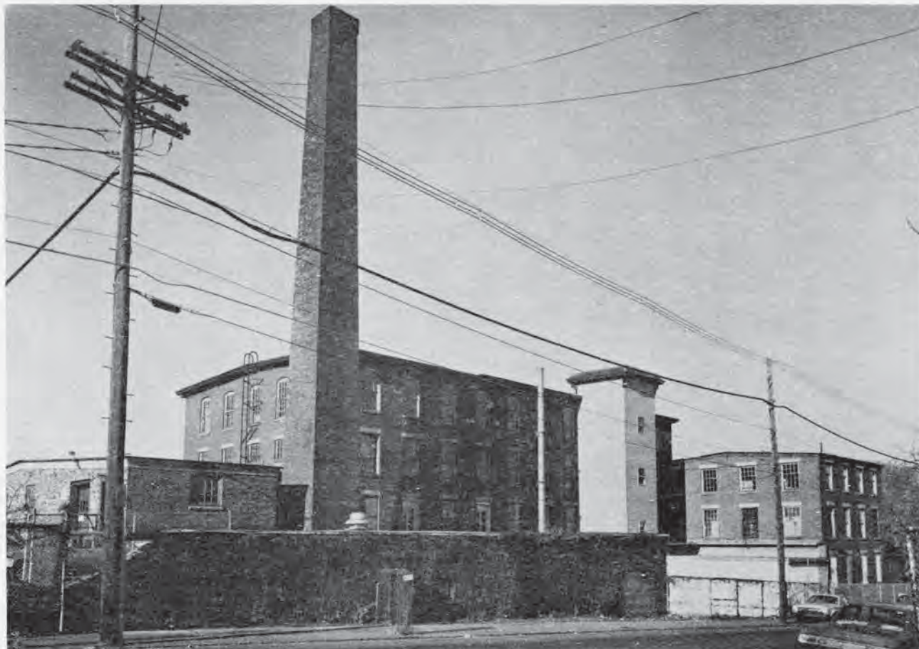
Figure 4-26 Belvidere No. 2 Mill, 645 Lawrence Street, built ca. 1863, photographed 1979.
