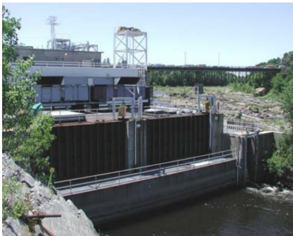
Figure 4.1-3. Fish lift entrance at the E.L. Field Powerhouse tailrace.
