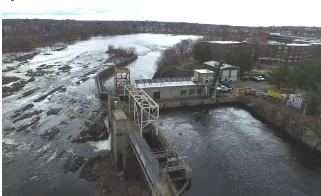
Figure 4.1-5. E.L. Field Powerhouse.
