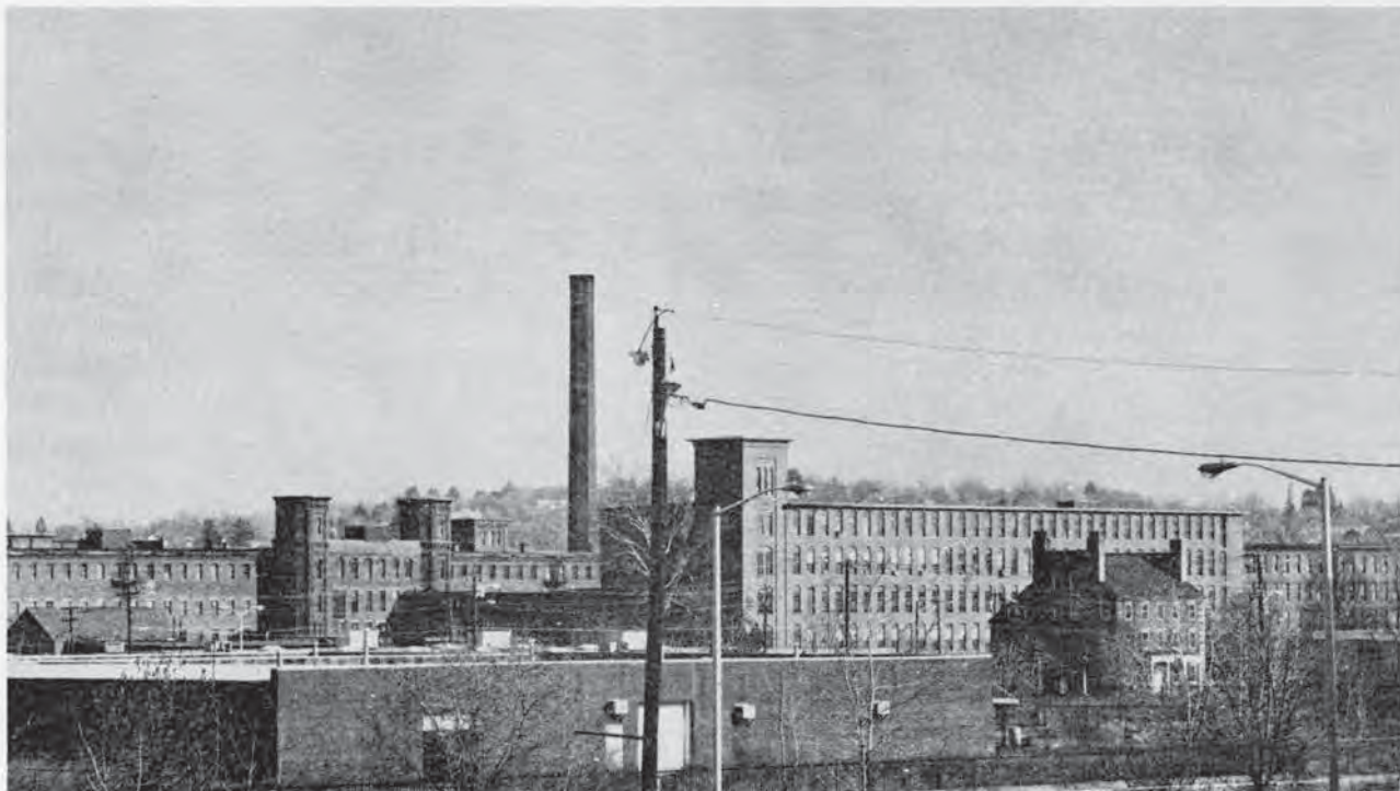
Figure 4-11 View of the Lawrence Manufacturing Company from the west, 1979.
