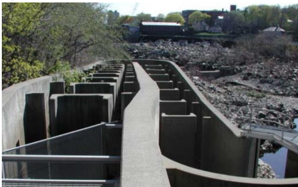
Figure 4.1-4. Fish Ladder at the Pawtucket Dam.
