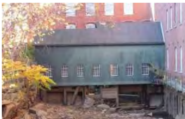
Boott Dam Gatehouse (DCR)
