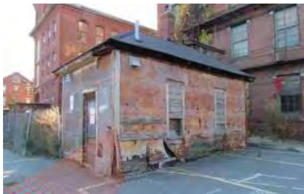
Hamilton Wasteway Gatehouse (DCR)
