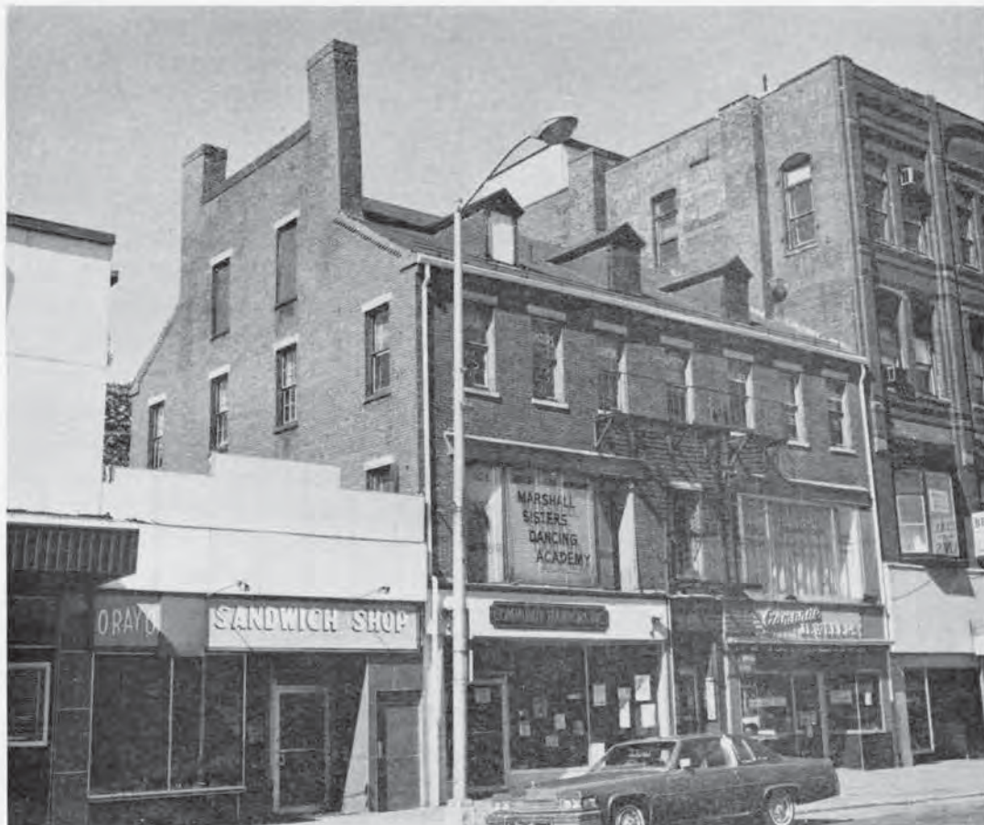
Figure 3-12 The Mansur Block, 101 Central Street, built ca. 1836, photographed 1979.
