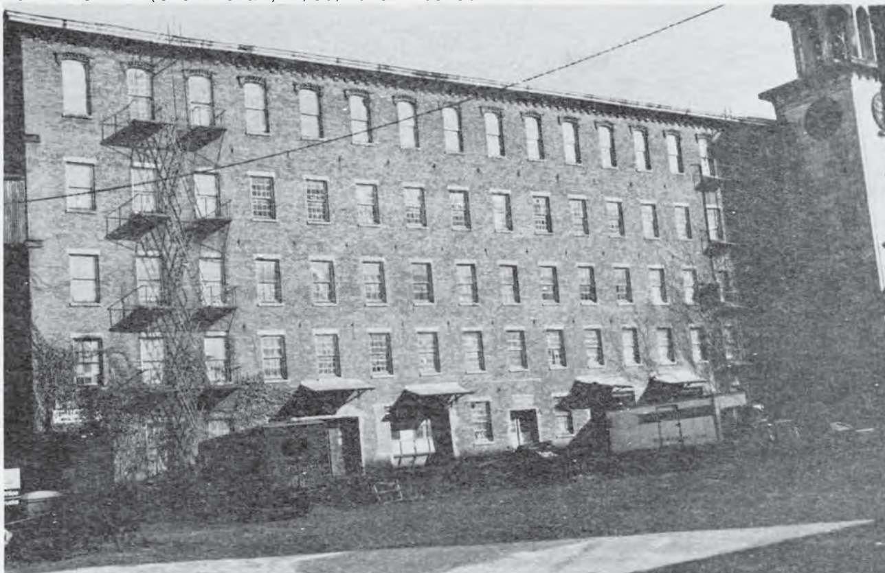
Figure 3-9 Mill No. 2, Boott Cotton Mills. Built 1835, top floor added ca. 1880, photographed 1979.
