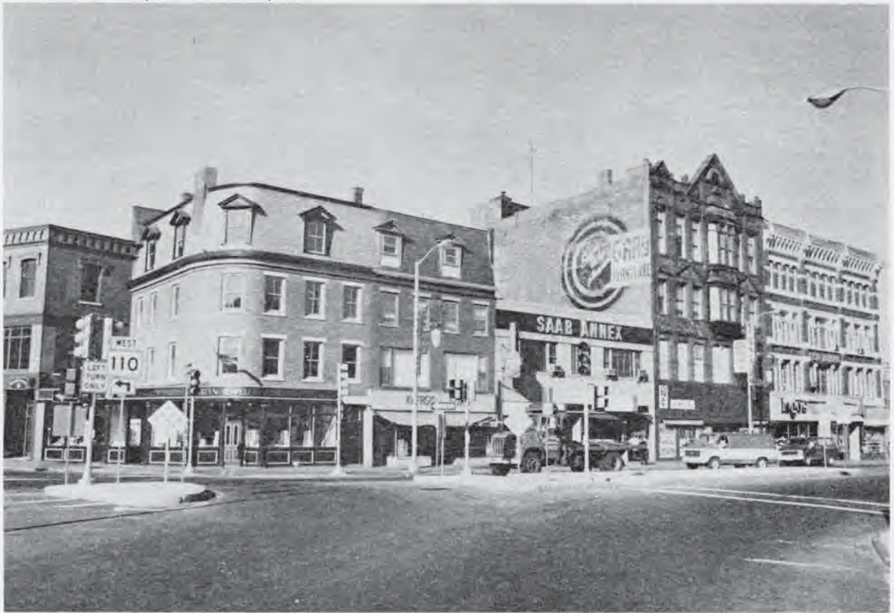
Figure 4-17 View of the Central Street block between Middlesex and Jackson Streets, 1979.
