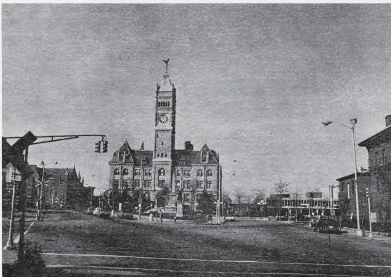
Figure 4-2 View of Monument Square from the east, 1979.
