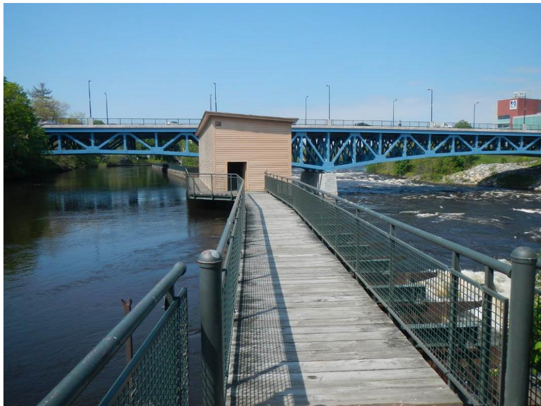
Figure 5.8-4. View looking upstream along the Northern Canal Walkway.
