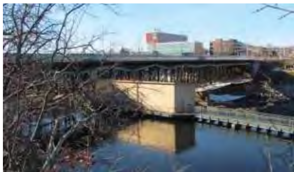
Northern Canal Wasteway Gatehouse (DCR)
