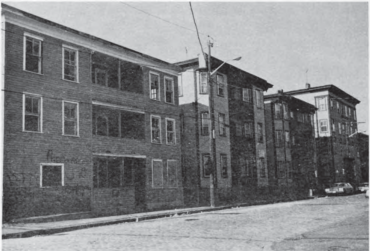
Figure 3-37 View of the west side of Adams Street, between Lagrange and Broadway Streets in the Acre neighborhood, November 1979.
