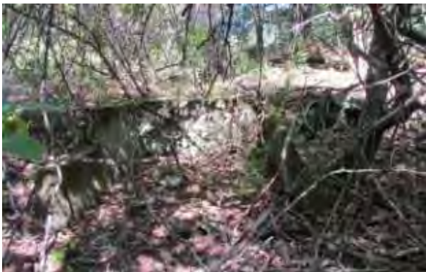
Outbuilding Foundation (DCR)
