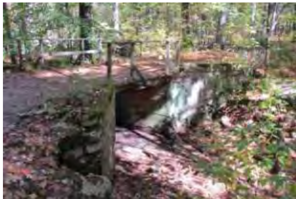
Small bridge on Woodchuck Trail (DCR)
