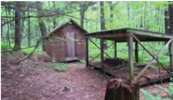
Cabin Shed and Lean-to (DCR)
