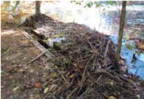
A culvert at the intersection of Woodchuck Trail and Garrison Loop. (DCR)
