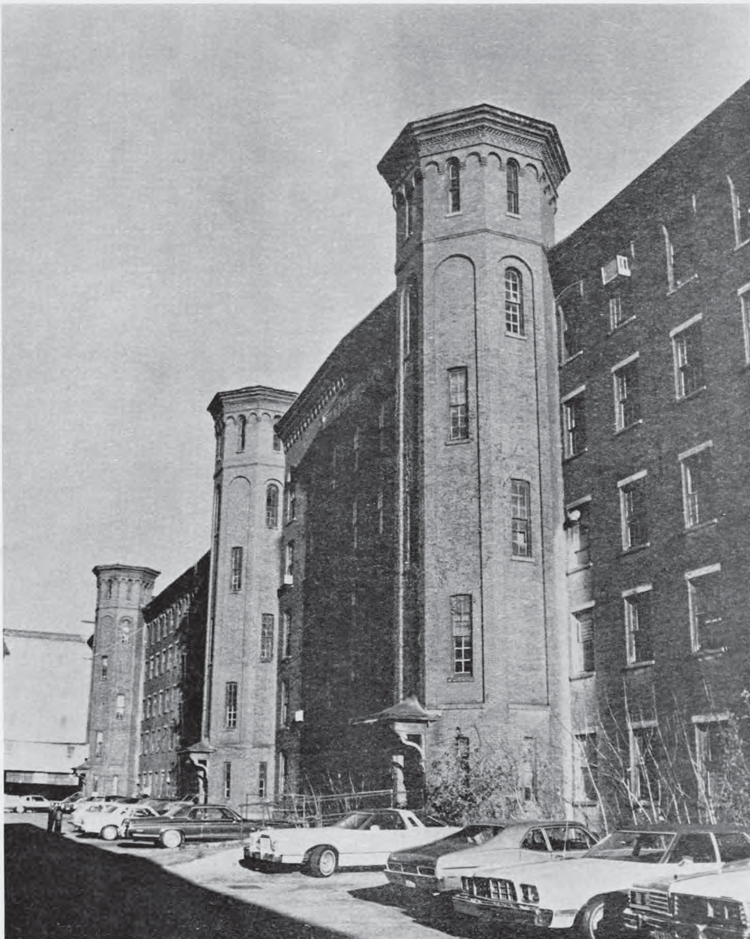
Figure 4-8 View of Mill No. 1, Massachusetts Cotton Mills, 1979. Right and left sections built 1839-40, center section 1862, left stair tower 1872.
