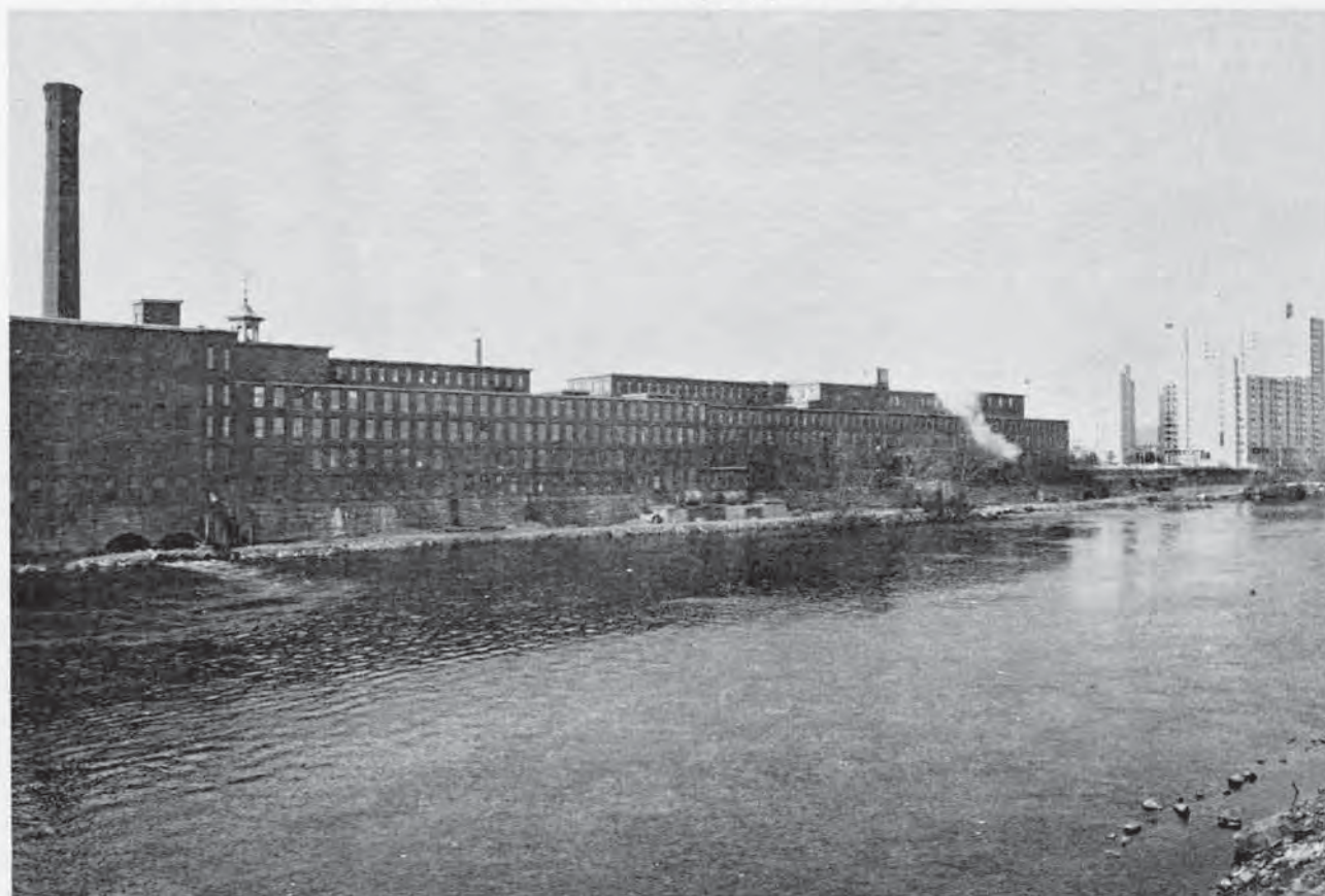
Figure 4-36 View from the east of the Boott Mills (left and center) and of the apartment towers on the site of the Merrimack Manufacturing Company (right), 1979.
