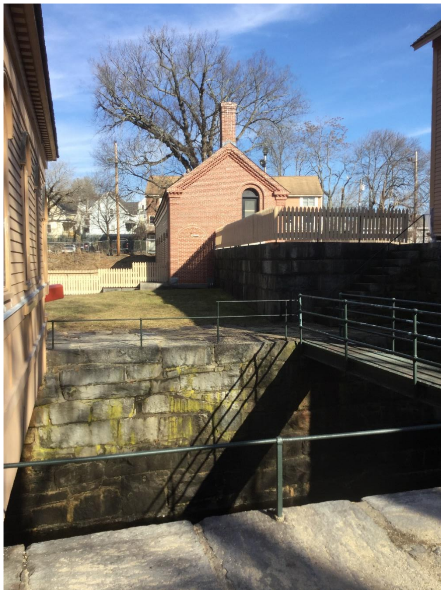
Figure 5.9-2. Guard Lock and Gates Facility.
