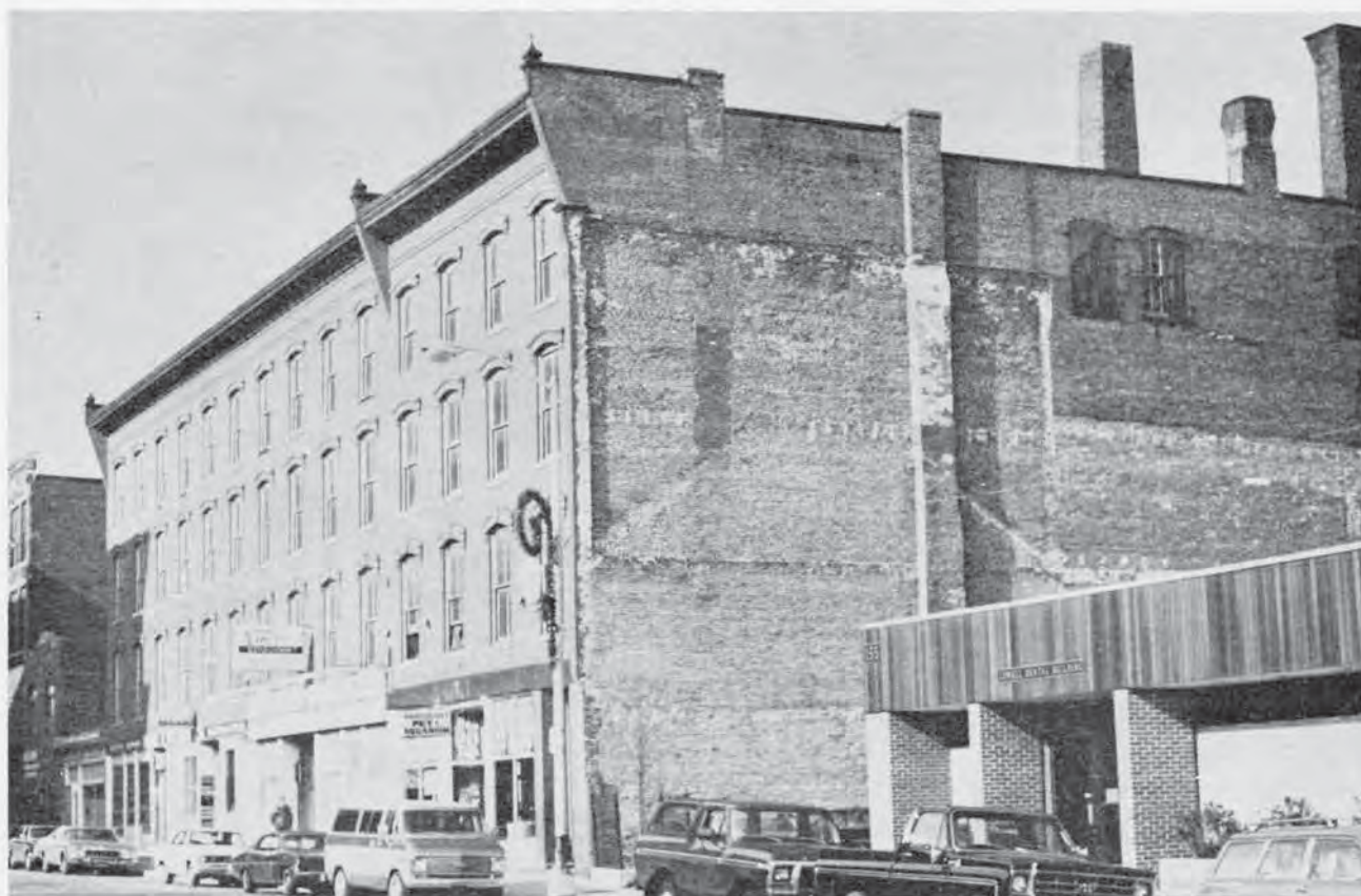
Figure 3-22 J. C. Ayer & Co. Building, 165 Market Street, built ca. 1858, photographed 1979.
