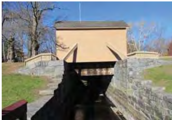
Great Gate and Gatehouse (DCR)
