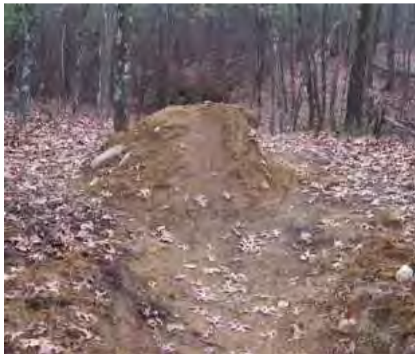
A mountain bike jump constructed in the forest. (DCR)
