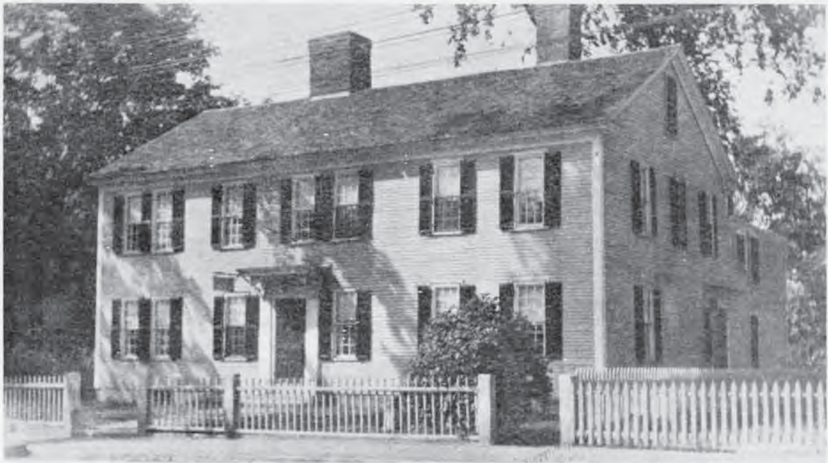
Figure 3-2 Spalding House, 383 Pawtucket Street, built 1761, photographed ca. 1920.
