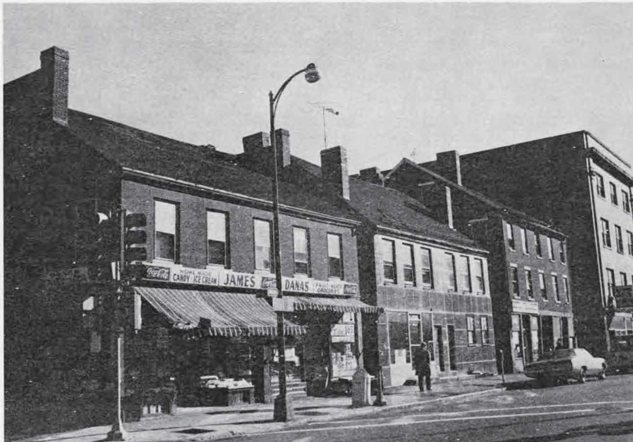
Figure 4-19 View of 62, 72, and 80 Gorham Street (left to right), all built ca. 1830, photographed 1979.
