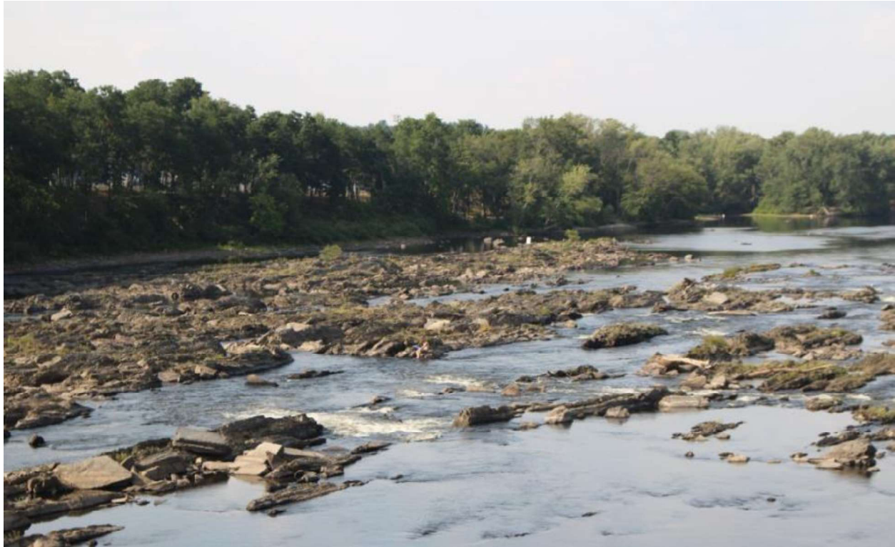
Fig. 1: Natural river channel dewatered by the Lowell Hydroelectric Project
