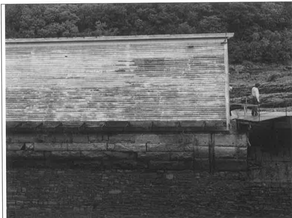
Photograph 5 – HAER Photograph MA-8C-2, taken in 1974 or 1975; note staining in wall and vegetation in joints below gatehouse, indicating that the normal elevation of the Northern Canal was several feet below what it is today. Also, note many open joints in larger masonry units at the top of the dam.
